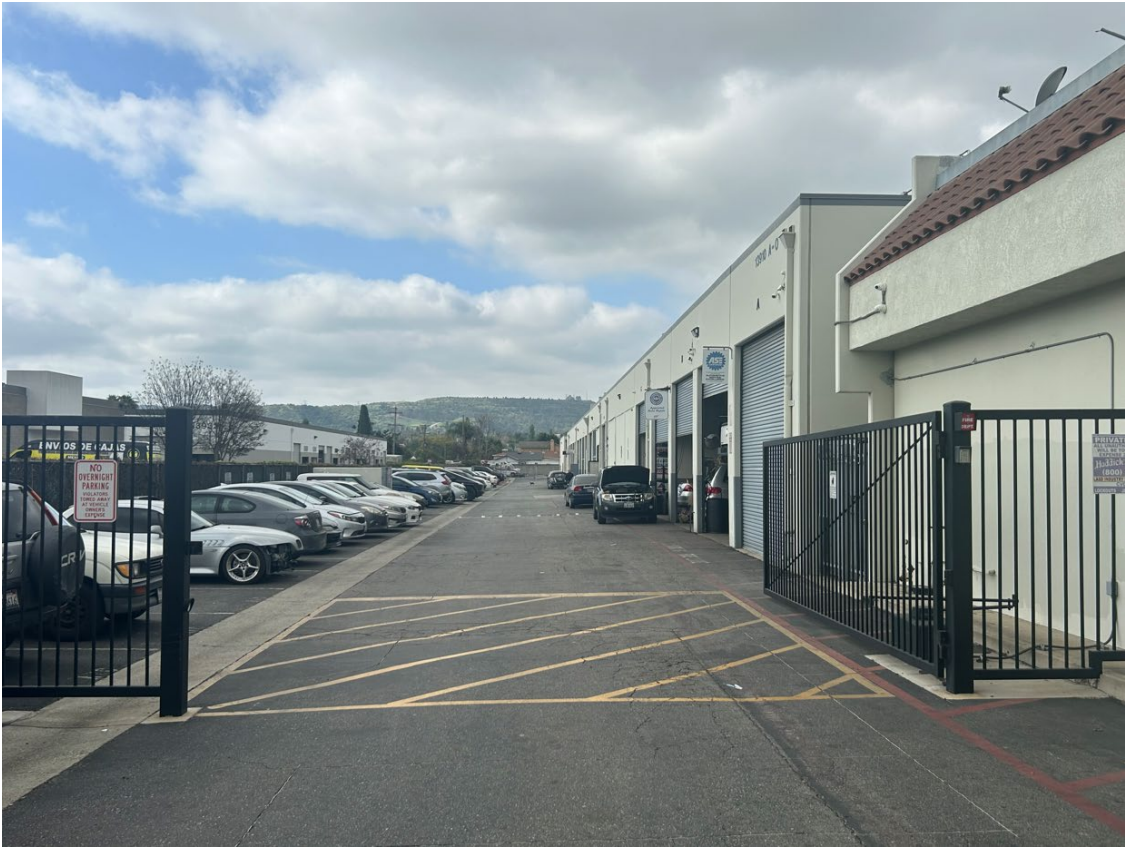
View of Auto Repair Industrial Building and Parking Spaces from the Northeast (Front)
