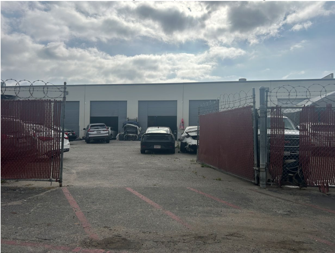
Exterior View of the Existing Auto Repair Industrial Building from the West
