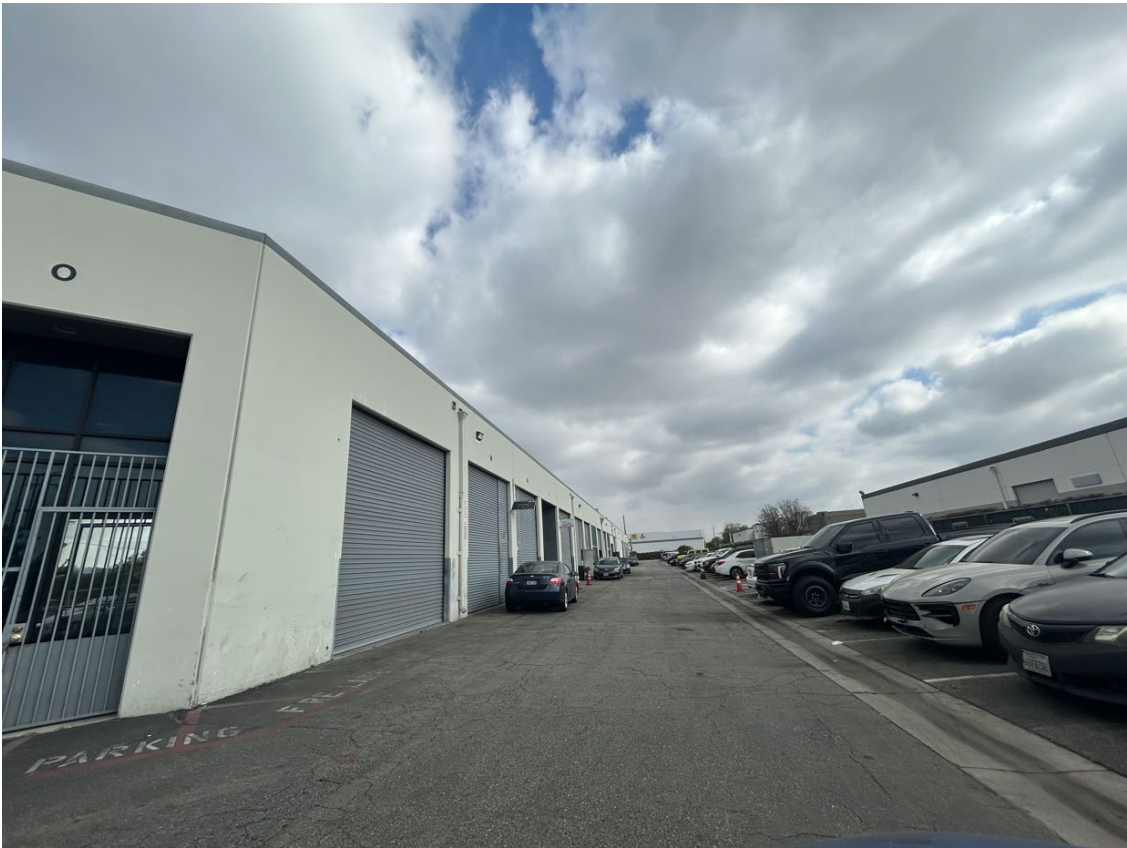
View of Auto Repair Industrial Building and Parking Spaces from the Southeast (Rear)
