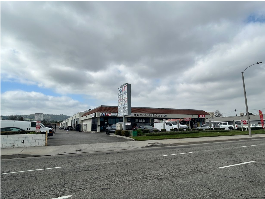
View of Subject Property from the Northeast (Front)
