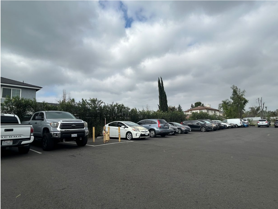
View of the Perimeter Wall at the South (Rear)
