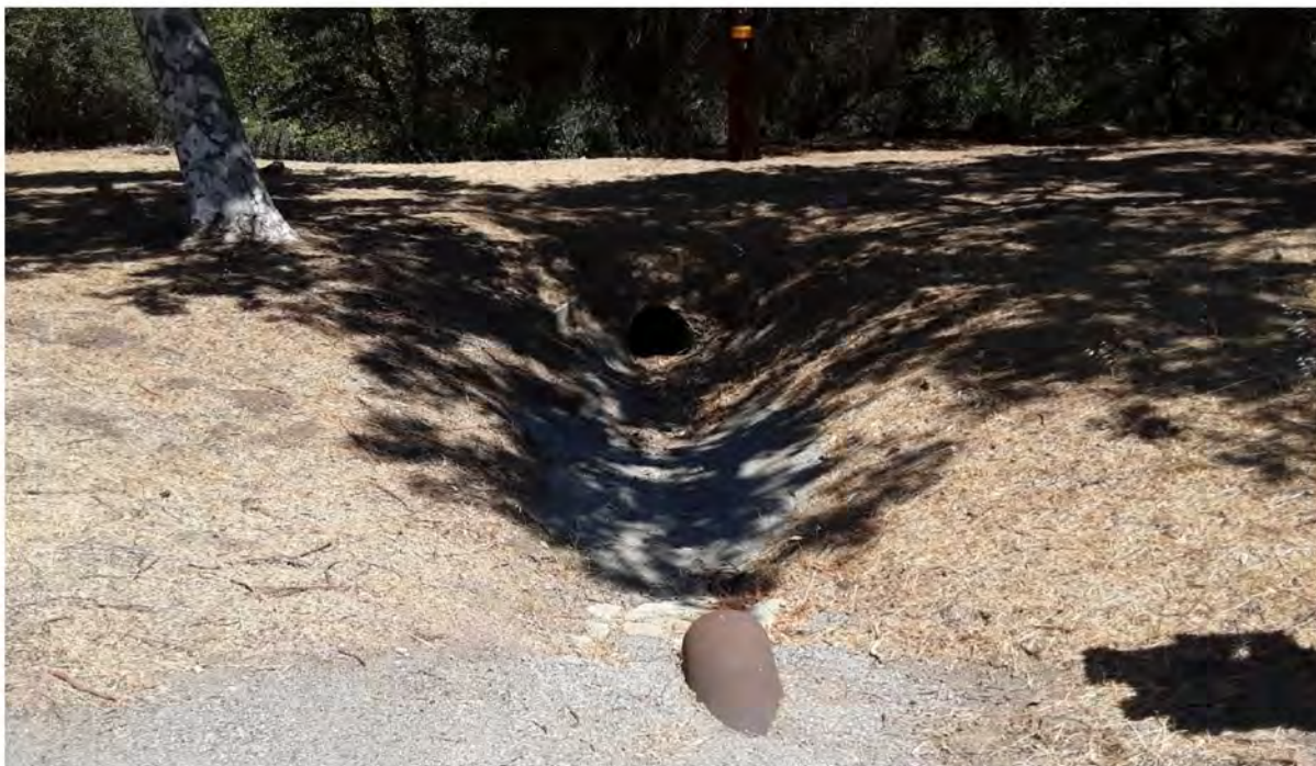
Photograph 6. Ephemeral ditch: outlet of culvert under Tapia WRF access road, concrete-lined ditch, and inlet of culvert that leads to Malibu Creek, facing north. Photo location 6. 7/21/2021
