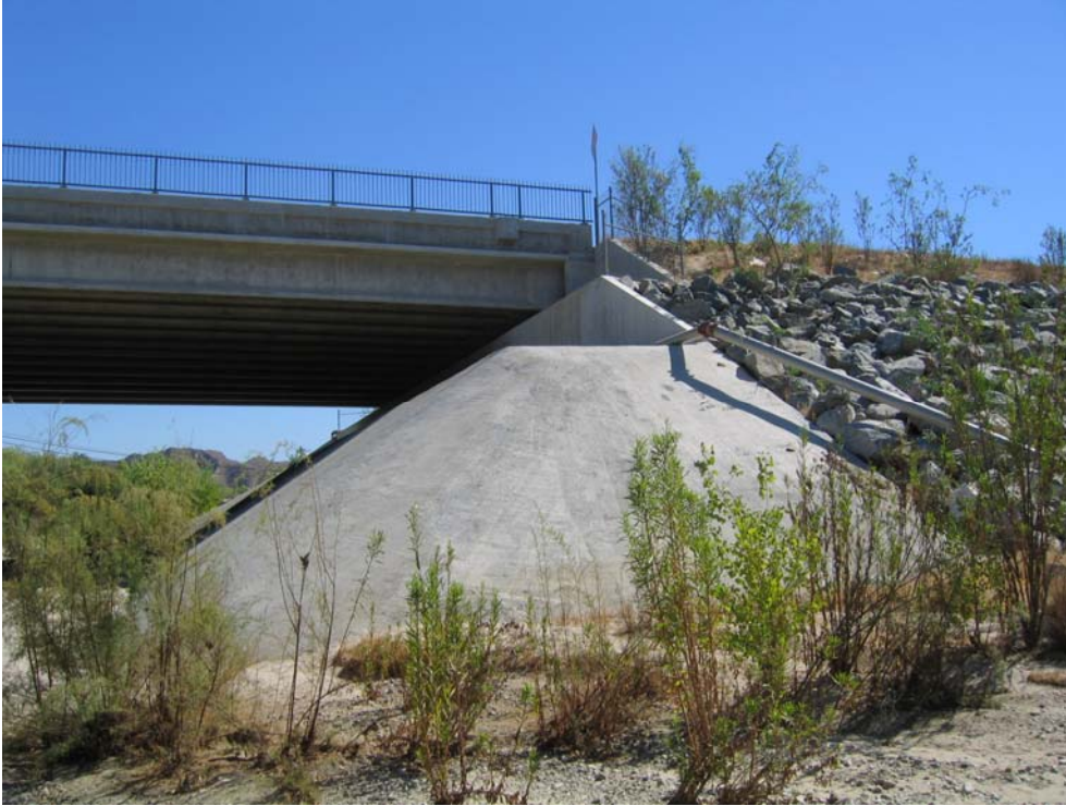
Photo 3. Commerce Ctr. Drive Bridge concrete abutment on the South side
