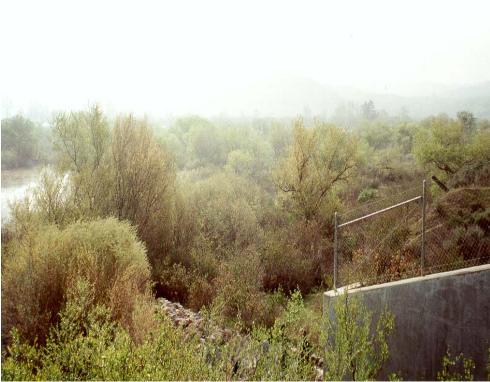
Photo 7. Vegetation at storm drain outlet for P.D. No. 2298
