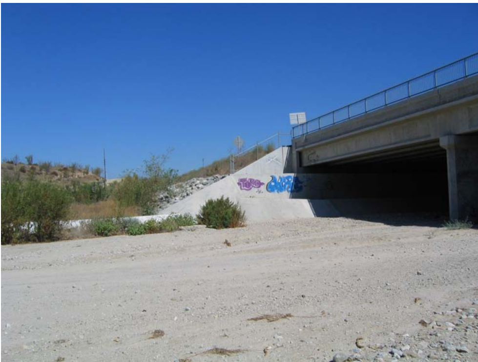
Photo 6. Downstream of Commerce Ctr. Drive Bridge looking North
