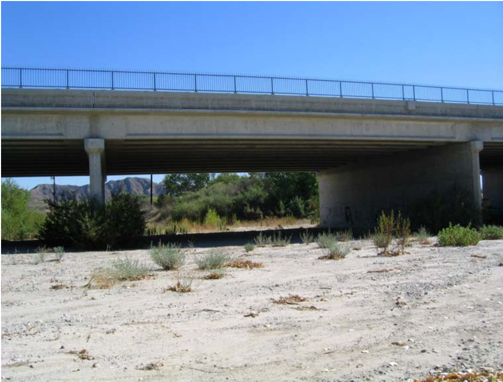
Photo 5. Downstream of Commerce Ctr. Drive Bridge looking upstream
