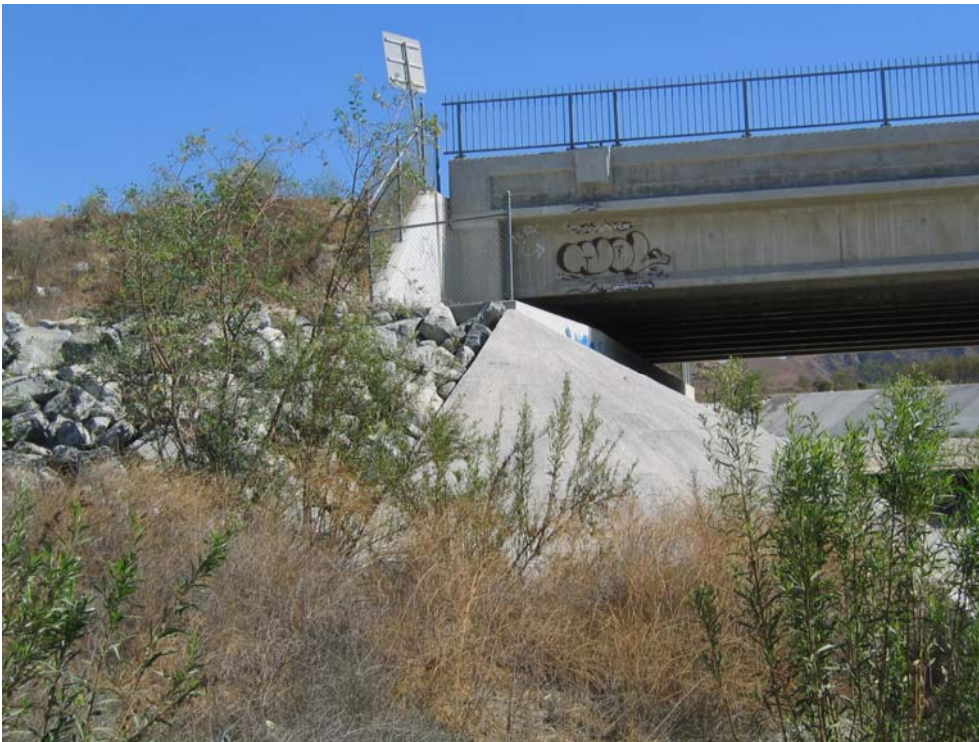
Photo 4. Commerce Ctr. Drive Bridge concrete abutment on the North side
