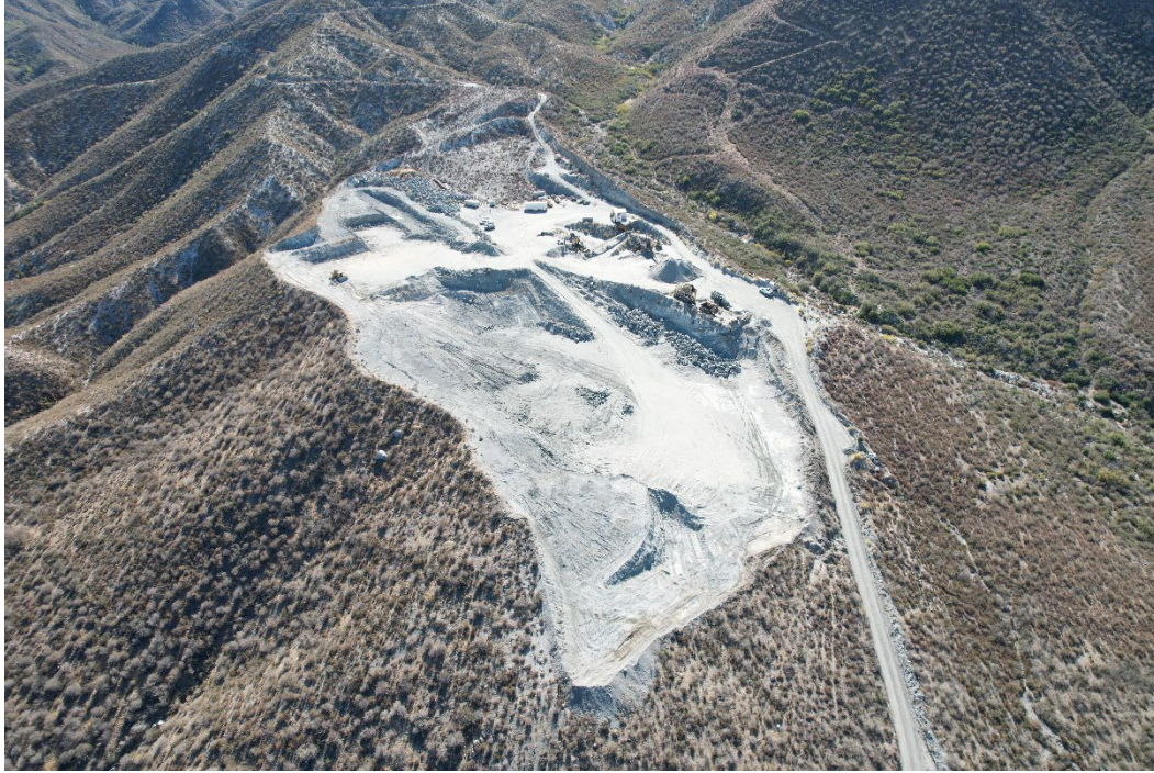
Photo #3-2021 Drone photo of Gray Quarry, looking south
