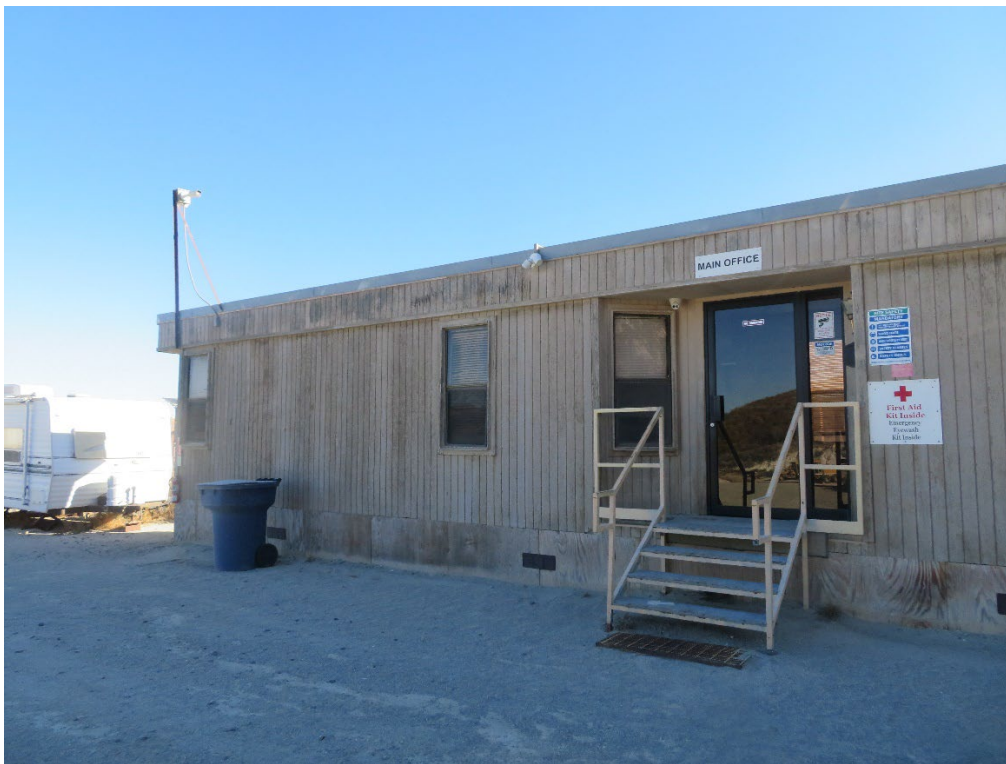
Photo #20-2025 photo of White Quarry office, looking east
