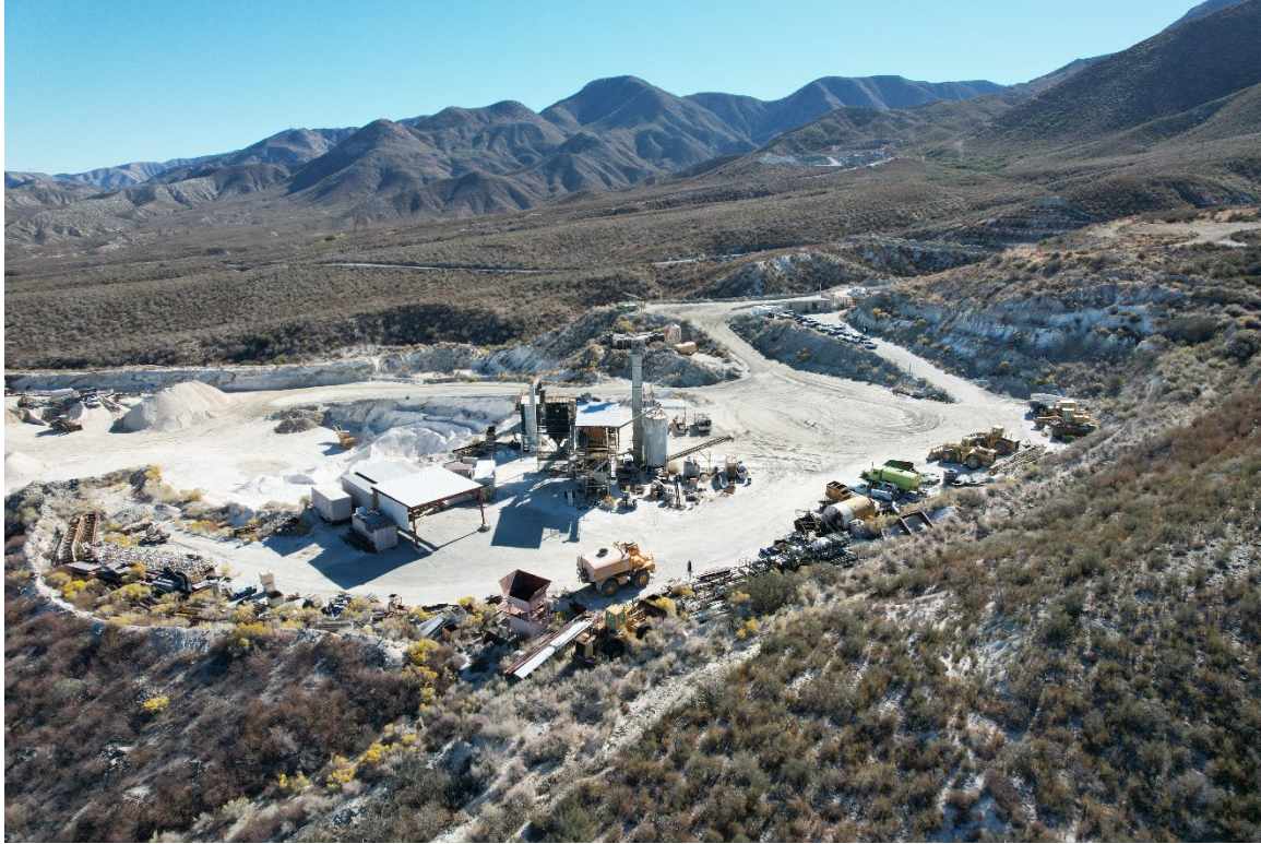
Photo #11-2021 Drone photo of White Quarry, looking east
