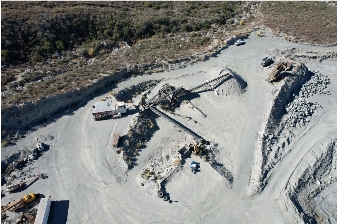
Photo #2-2021 Drone photo of Gray Quarry, looking west
