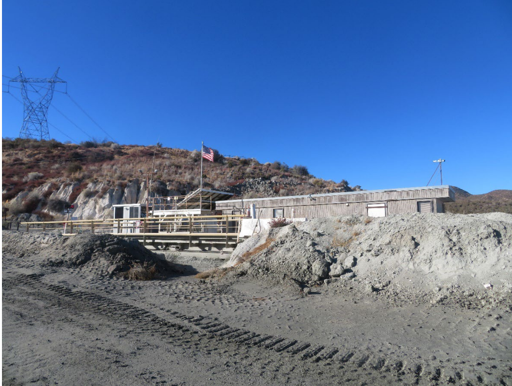
Photo #17-2025 photo of White Quarry scale house & office, looking west
