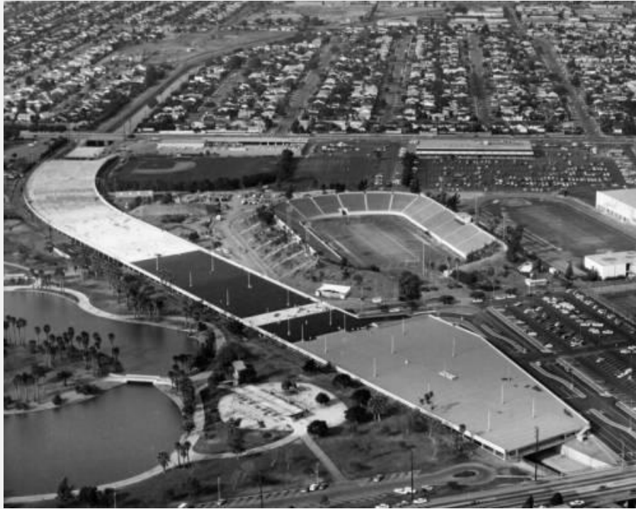
Exhibit 1. Aerial photograph of El Camino College and the surrounding community (undated).
