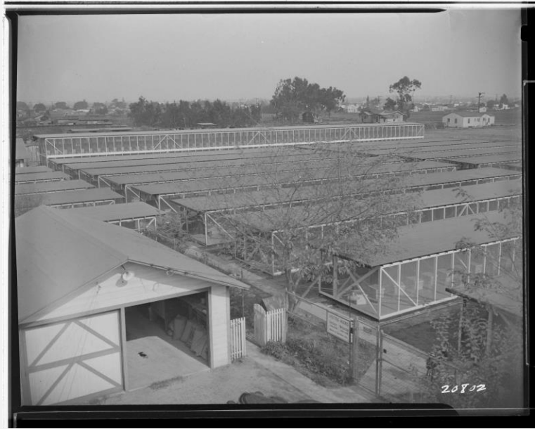
Exhibit 9. Chapman Chinchilla Farm, which was located at 4957 West 104th Street in Lennox, 1937.
