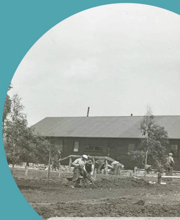
Alondra Park under construction, 1935
