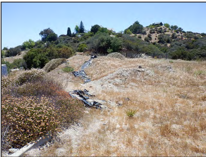
Photo 3 – The small stockpile of undocumented fill at the graded pad is shown. View faces southwest.
