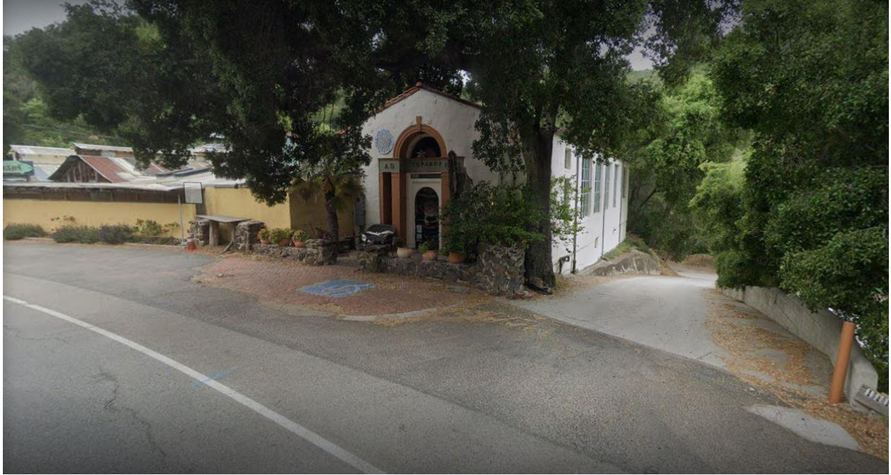
1105 N TOPANGA CANYON BLVD DRIVEWAY VIEW
