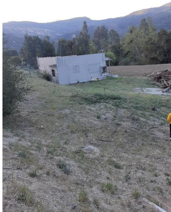
View to SE from NW corner of site
