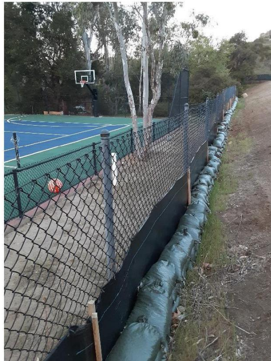
View to w along S fence
