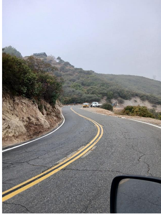
View to northwest at east end of site
