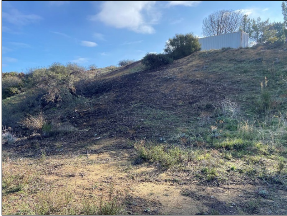
Photo 1. South slope leading up to zone A, facing northeast
