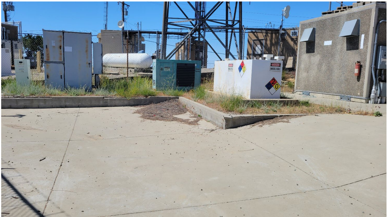
View of south property line and existing equipment (from left to right: 2 utility cabinets, backup generator, fuel tank, and equipment shelter). WCF in the background (behind the chain-link fence) is on a separate parcel and not part of this project.
