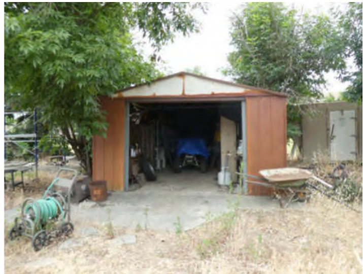
Photo #14: Metal shed located west of the dwelling
