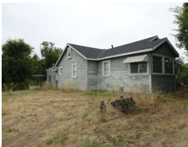
Photo #11: Dwelling at northeast corner (view from southeast)
