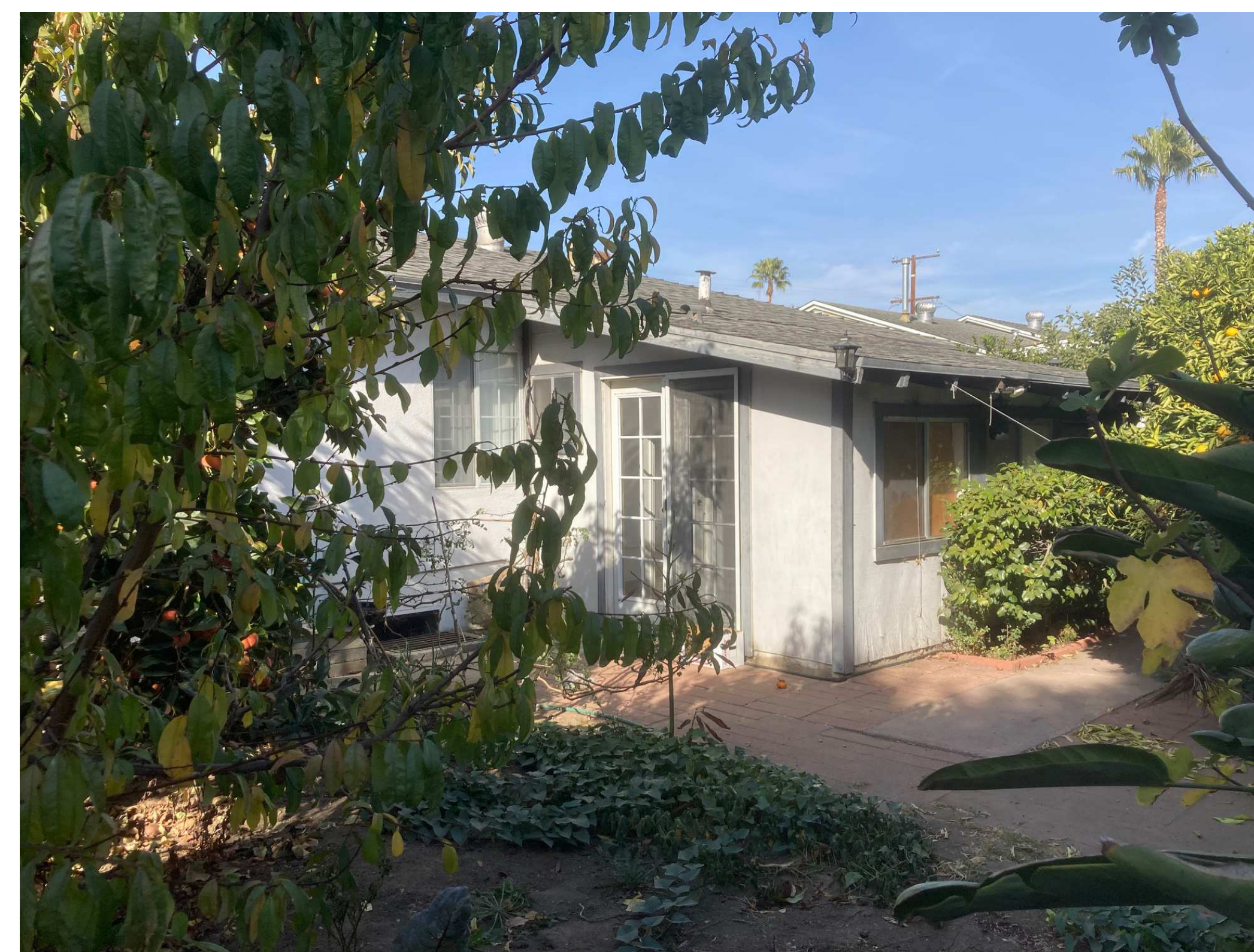
REAR YARD VIEW LOOKING NORTH
