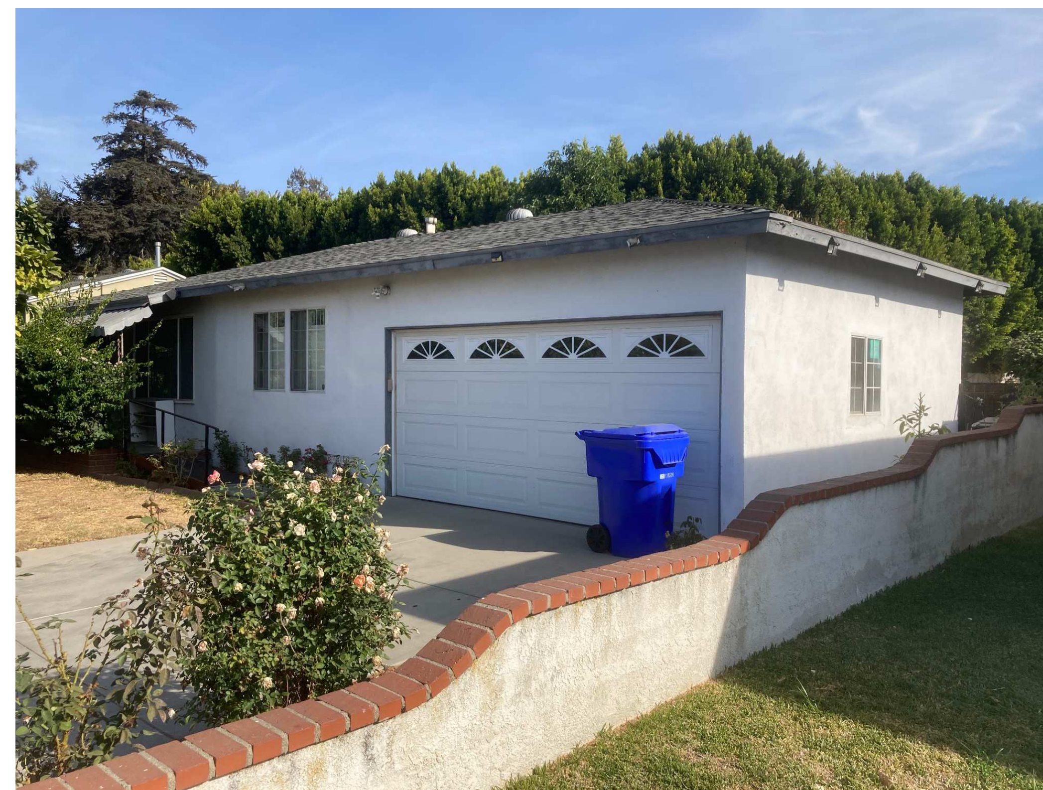
STREET VIEW LOOKING WEST
