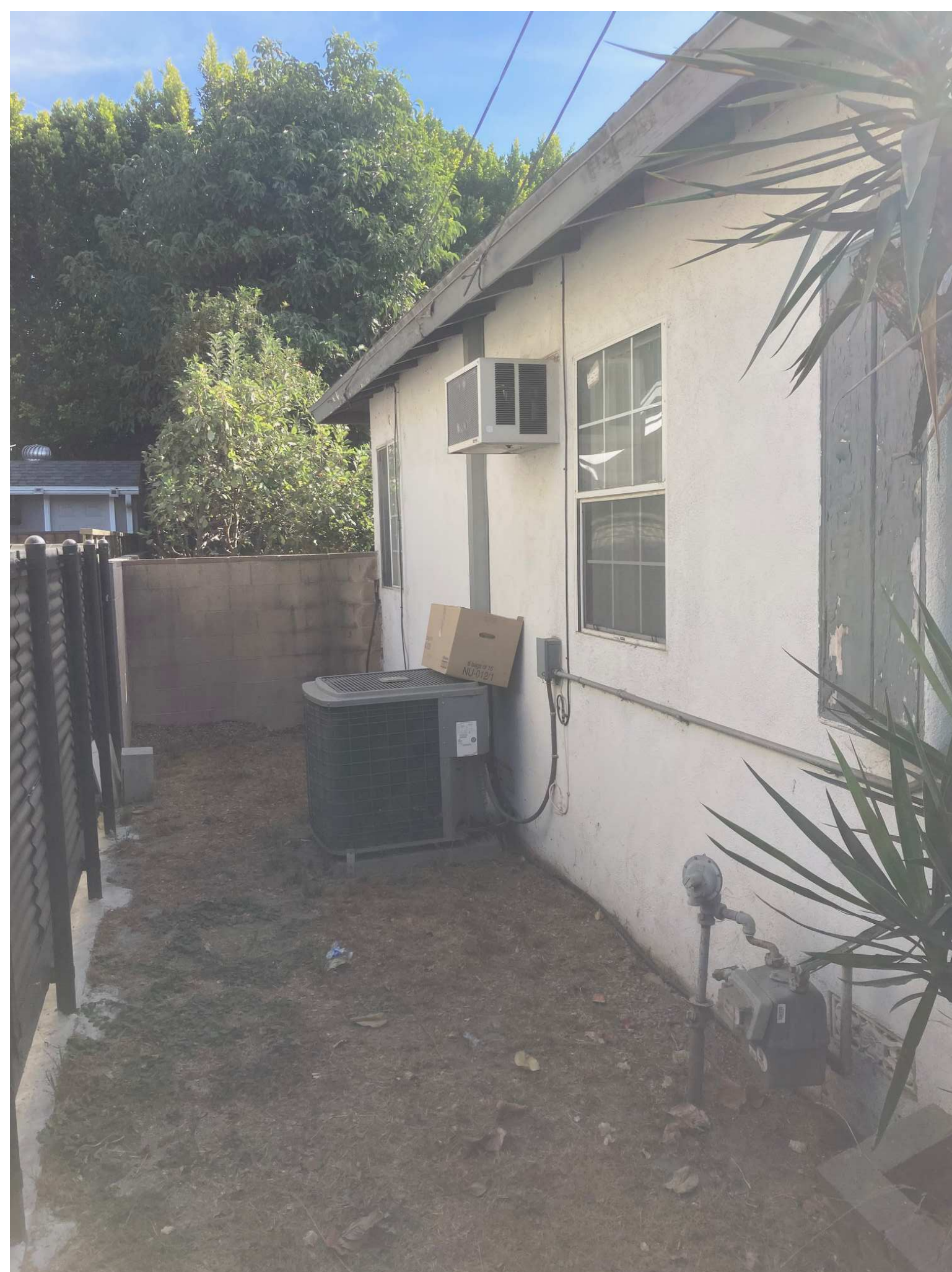
NORTH SIDE YARD
