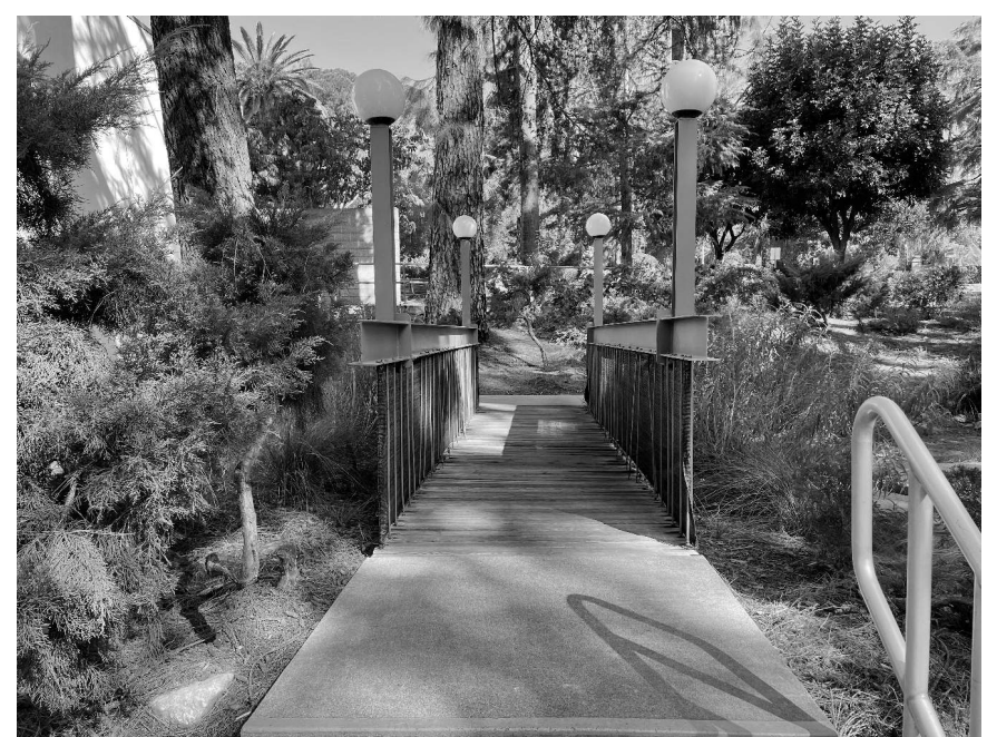
SANTA ROSA FOOTBRIDGE PHOTOS
