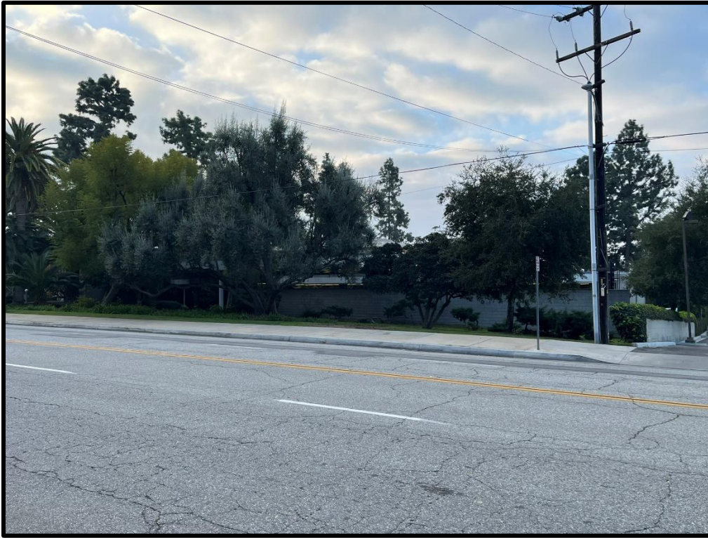
North elevation, west and central portion, facing south. New entrance door and parking lot planned for west portion of the elevation, potential sunken amphitheater planned for central portion; several trees will be removed.
