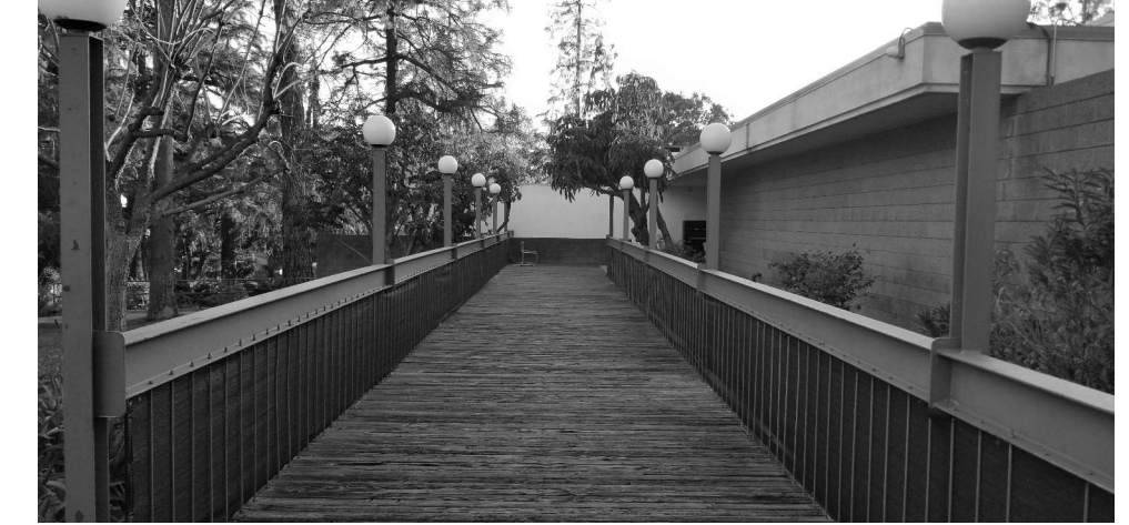
E MARIPOSA FOOTBRIDGE PHOTOS
