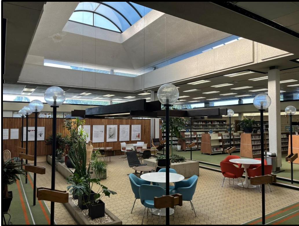
Sunken reading area, facing southwest. Steps on left side of image will be replaced with ADA-compliant ramp, globe lamps will remain. Portion of wood wall on left side of image will be removed.
