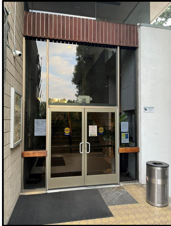
South elevation entry doors. These will be removed.
