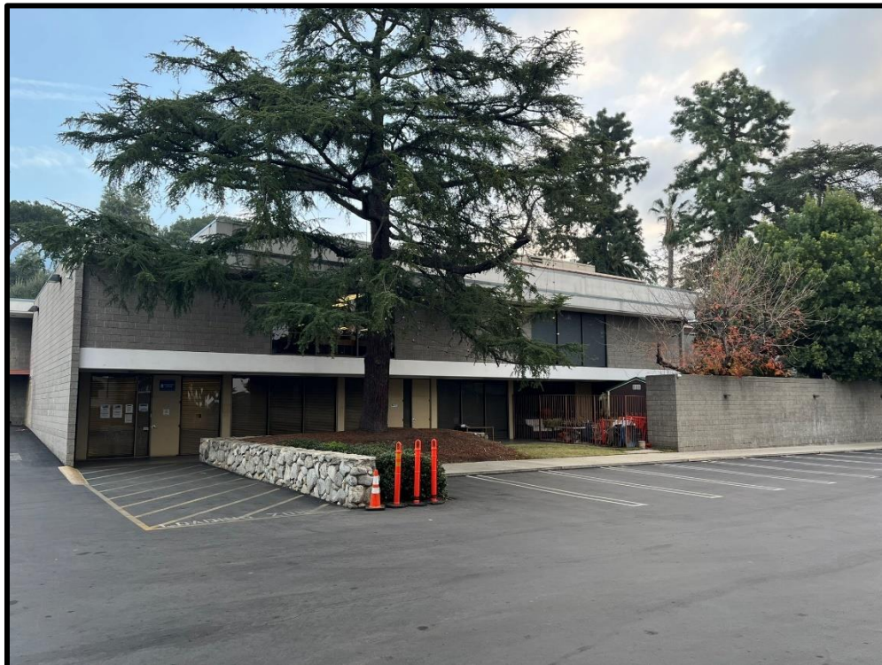
South elevation, facing northeast. Doors and fenestration on first floor will be altered.
