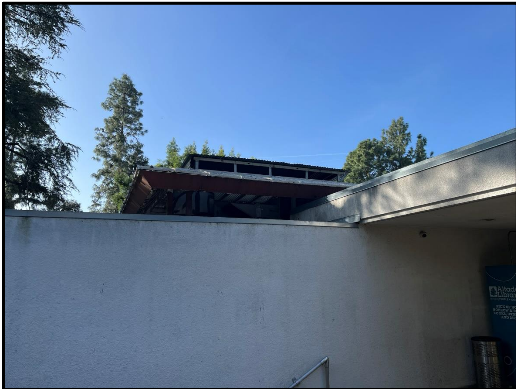
HVAC enclosure. Modifications will be made to make them more cohesive with the building.
