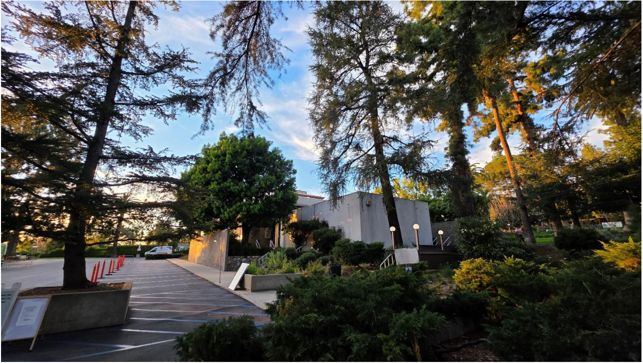
Existing Altadena Main Library entrance at Santa Rosa Avenue
