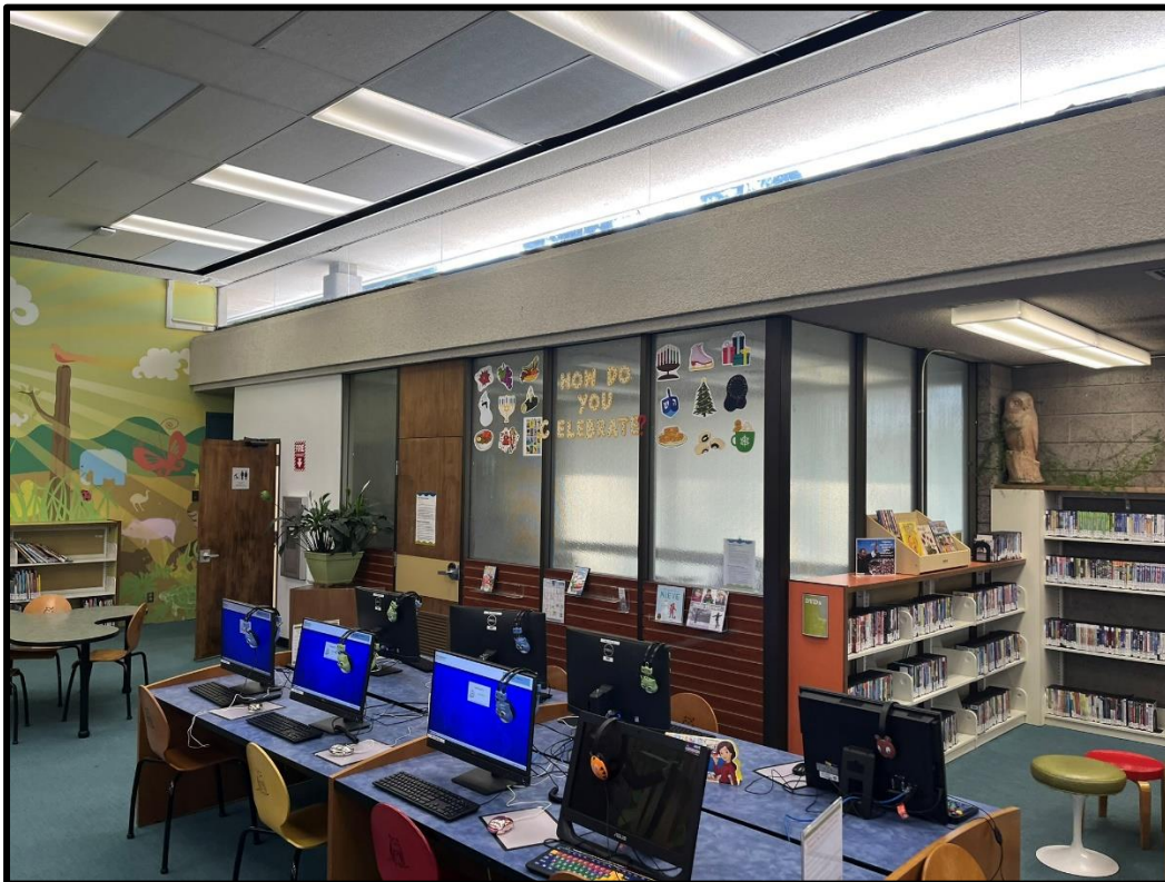
Western portion of main floor, facing southeast. New lobby area will be constructed here.
