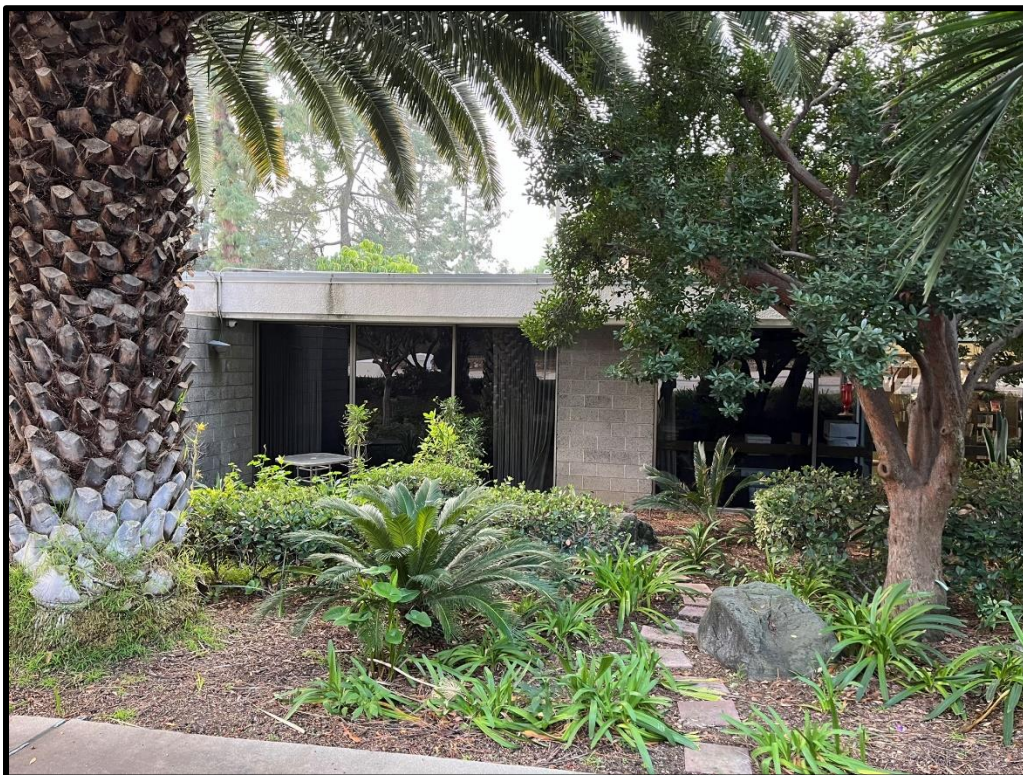
North elevation, east portion, facing south. Fenestration and doors will change.
