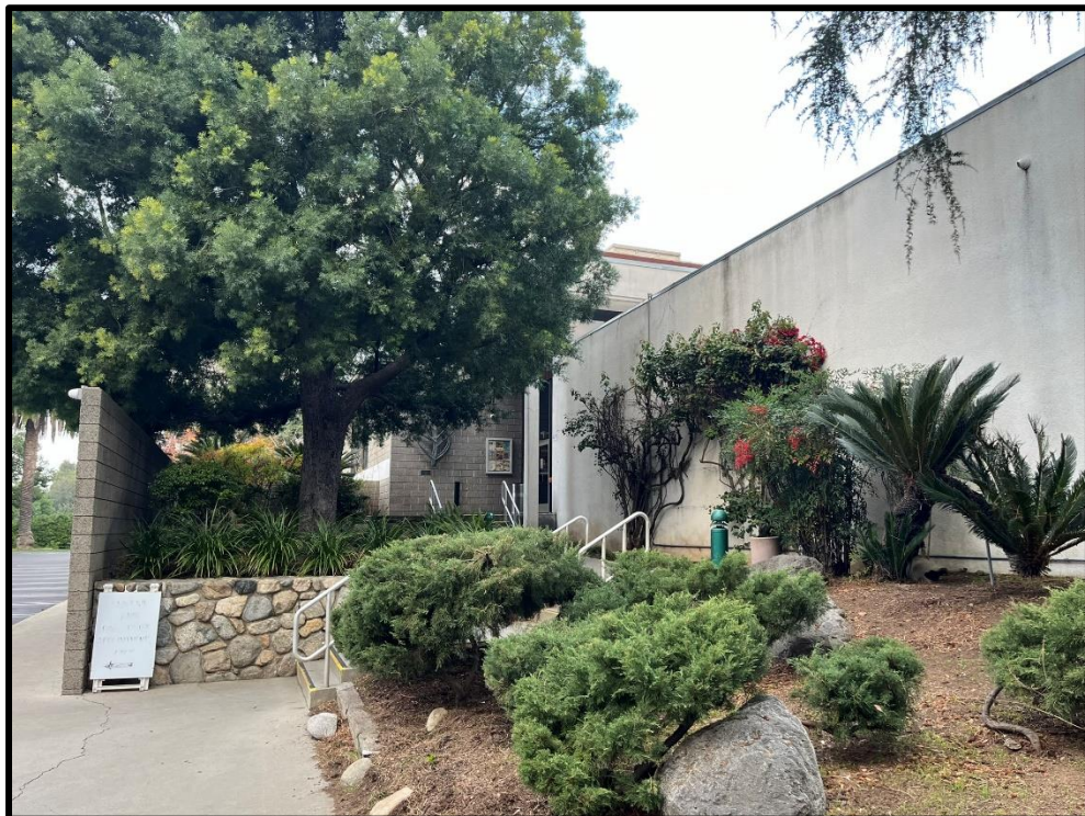
South and east elevations, facing northwest. New two-story atrium/entrance and deck will be located on this elevation.
