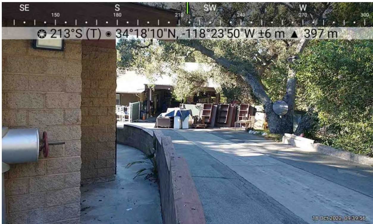
Image 5. Depicts the existing building and driveway on the south end of the project site.
