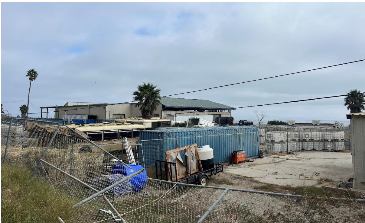
Photograph 8. View of developed area within the proposed project site. View facing northeast. October 9, 2023.
