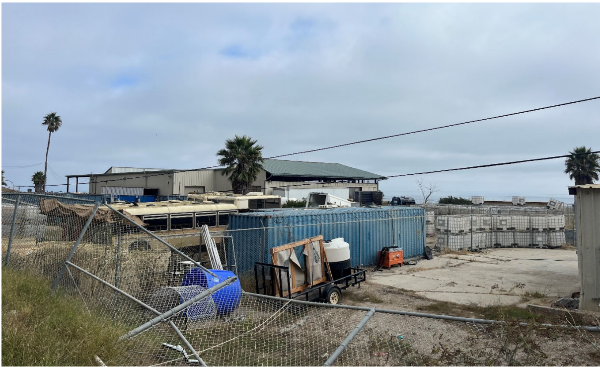
Photograph 8. View of developed area within the proposed project site. View facing northeast. October 9, 2023.
