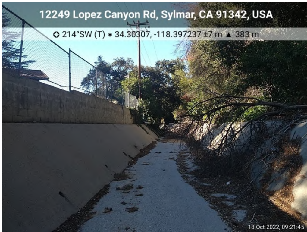
Photo 12. View of unnamed ephemeral channel #1 from its OHWM bounds, facing southwest.
