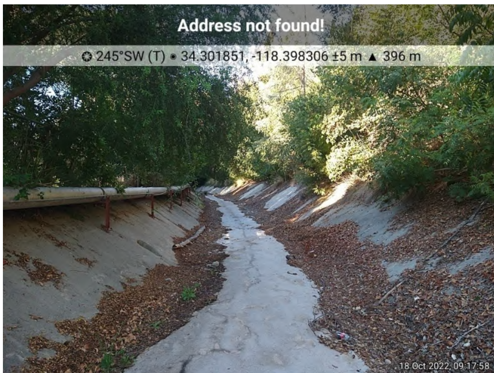
Photo 2. View of unnamed ephemeral channel #1 from its OHWM bounds, facing southwest.
