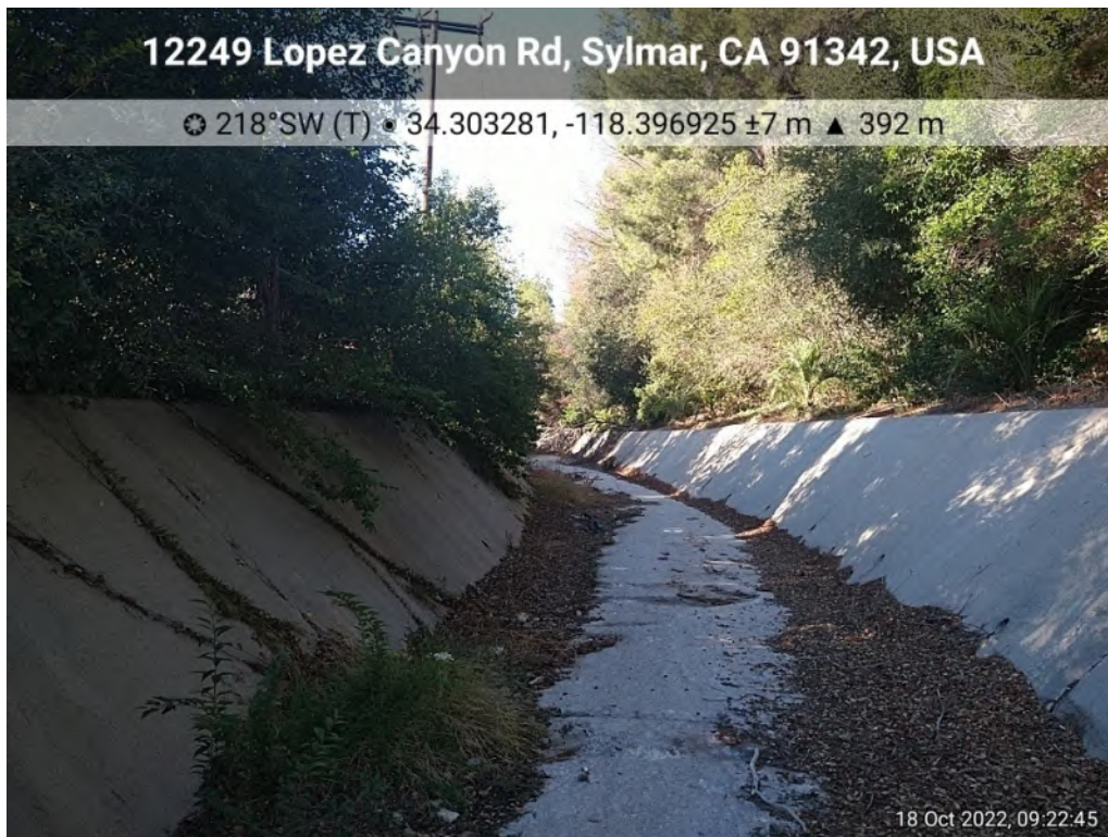
Photo 14. View of unnamed ephemeral channel #1 from its OHWM bounds, facing southwest.
