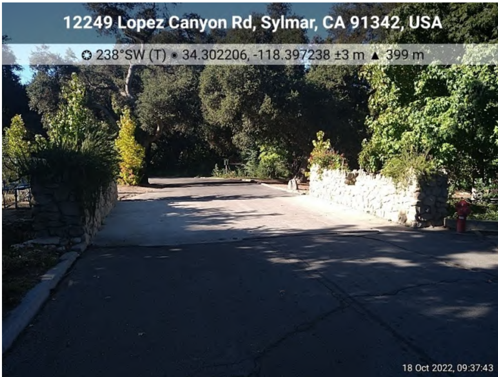
Photo 25. View of the property driveway to be re-paved in the proposed development, facing south. Unnamed ephemeral channel traverses under the bridge from left to right.
