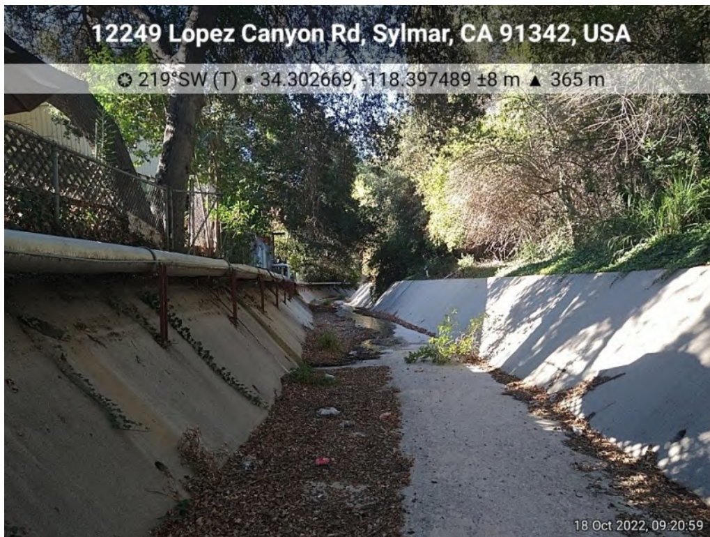
Photo 10. View of unnamed ephemeral channel #1 from its OHWM bounds, facing southwest.
