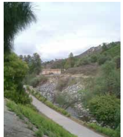
Example of multi-use path in a drainage channel.
