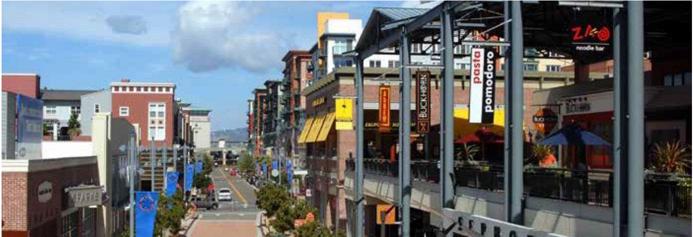
Example of TOD adjacent to Emeryville, CA transit station.
