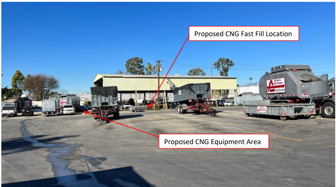
Photograph 4 - The CNG fueling equipment area will be located in front of the metal canopy structure.
