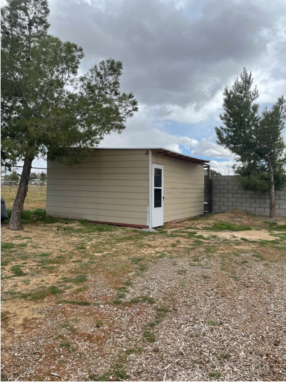
View of existing shed on southerly side yard:
