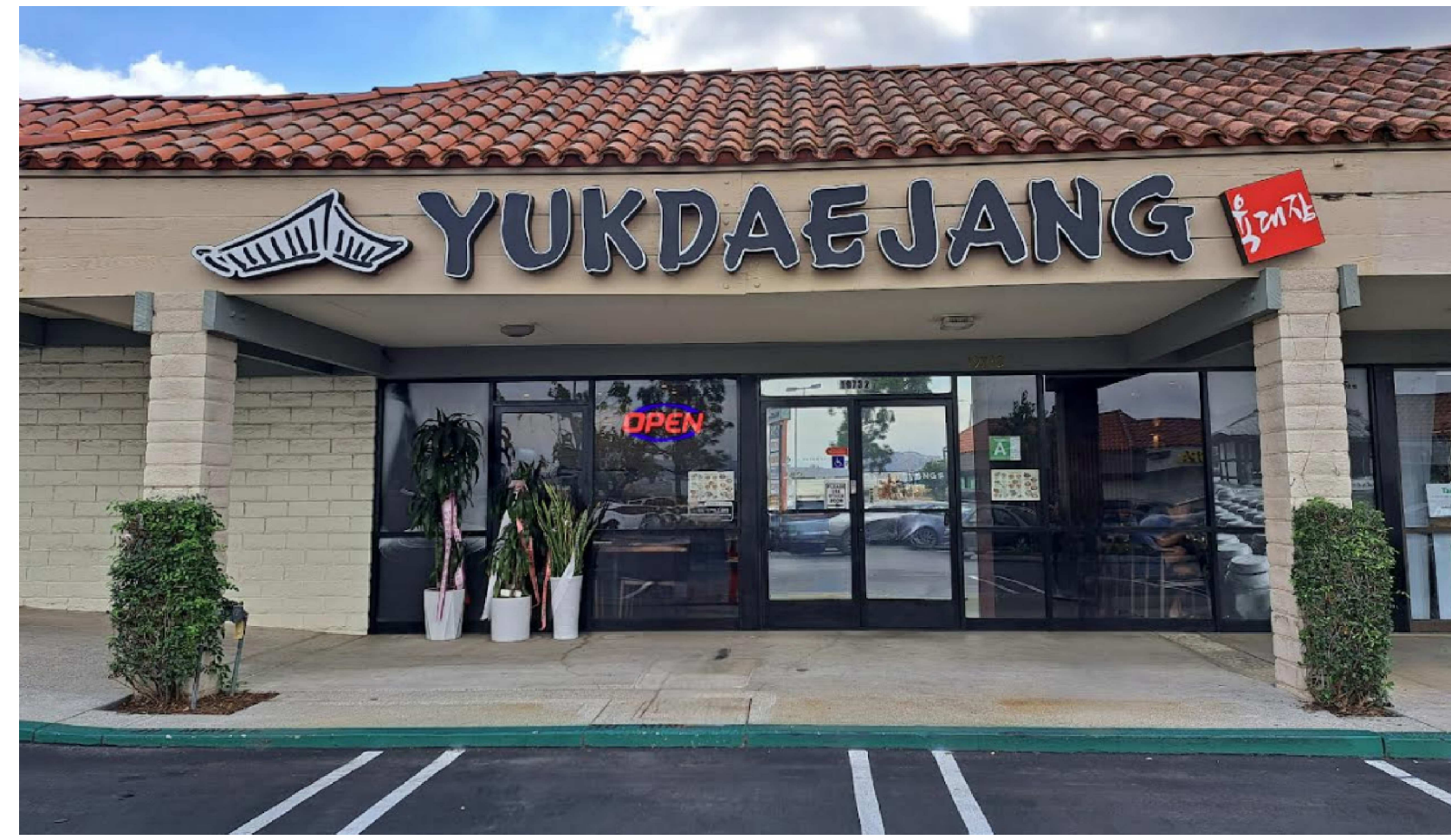
2 EXISTING RESTAURANT FRONT VIEW SCALE: NTS
