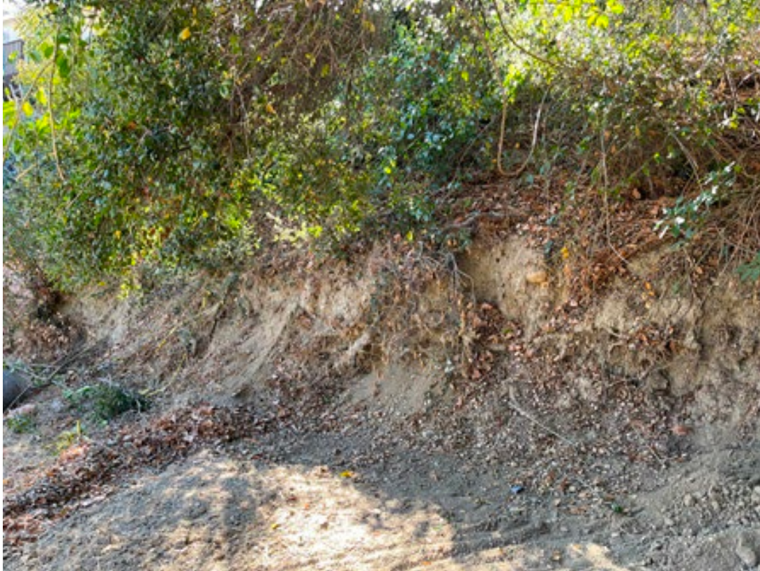
Cut slope at the south edge of the subject property.
