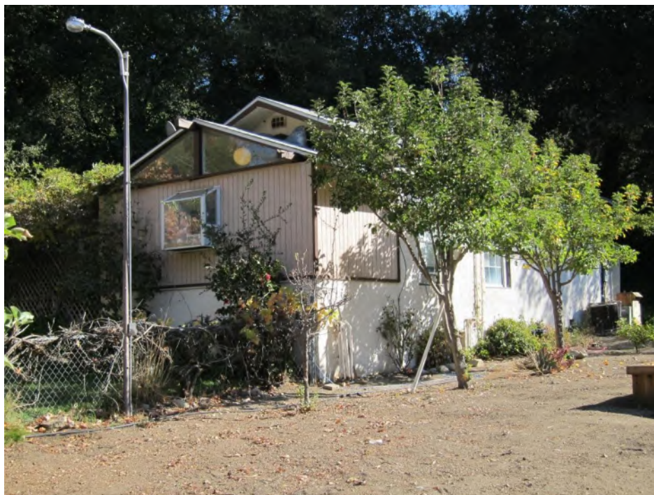
Photograph 8. Overview of altered cottage north and west elevations, view to southeast
