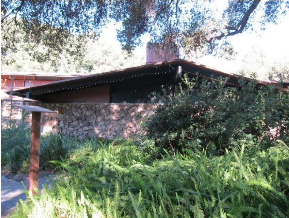
Photograph 14. South elevation, view to north
