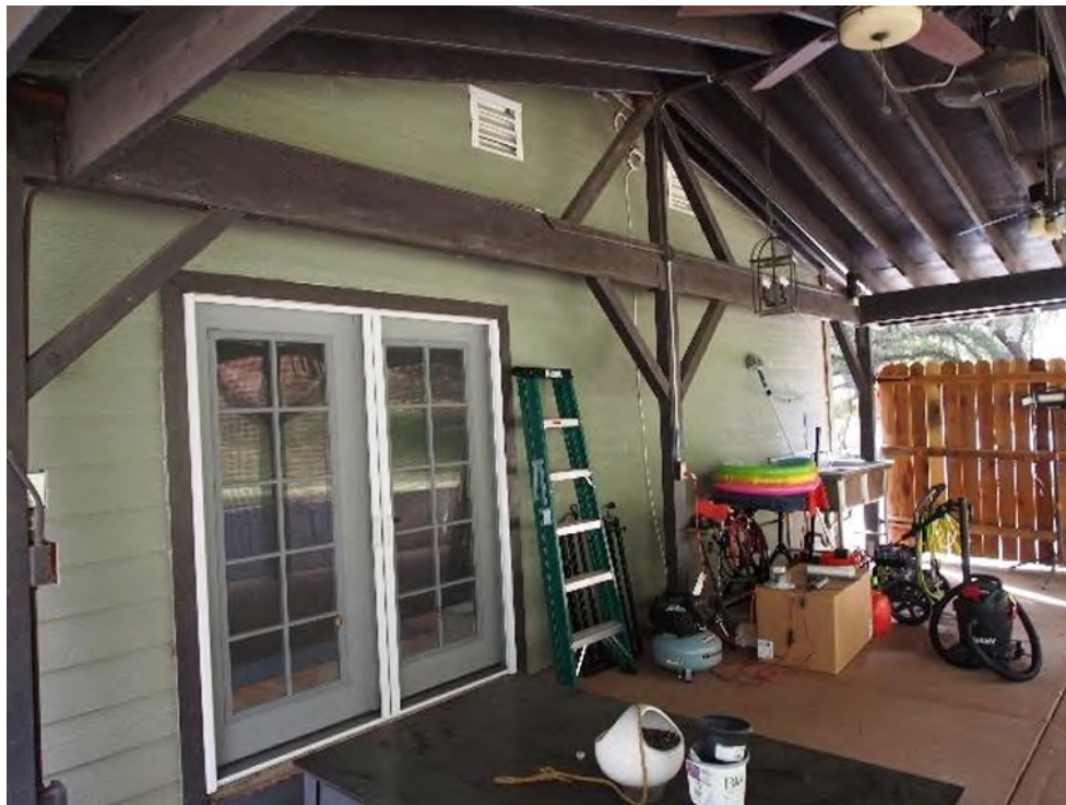
Photograph 37. Rear (north) elevation showing French doors and shade structure, view to southwest
