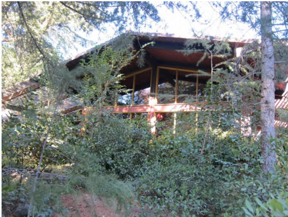
Photograph 2. Overview of window wall on south elevation, view to north
