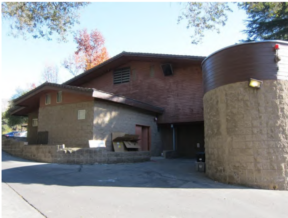
Photograph 4. Overview of rear (west) elevation showing extensive use of split-face CMU, view to east
