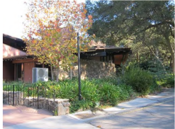
Photographs (from top): South elevation, view to northeast; South elevation, view to north; West elevation, view to east.
