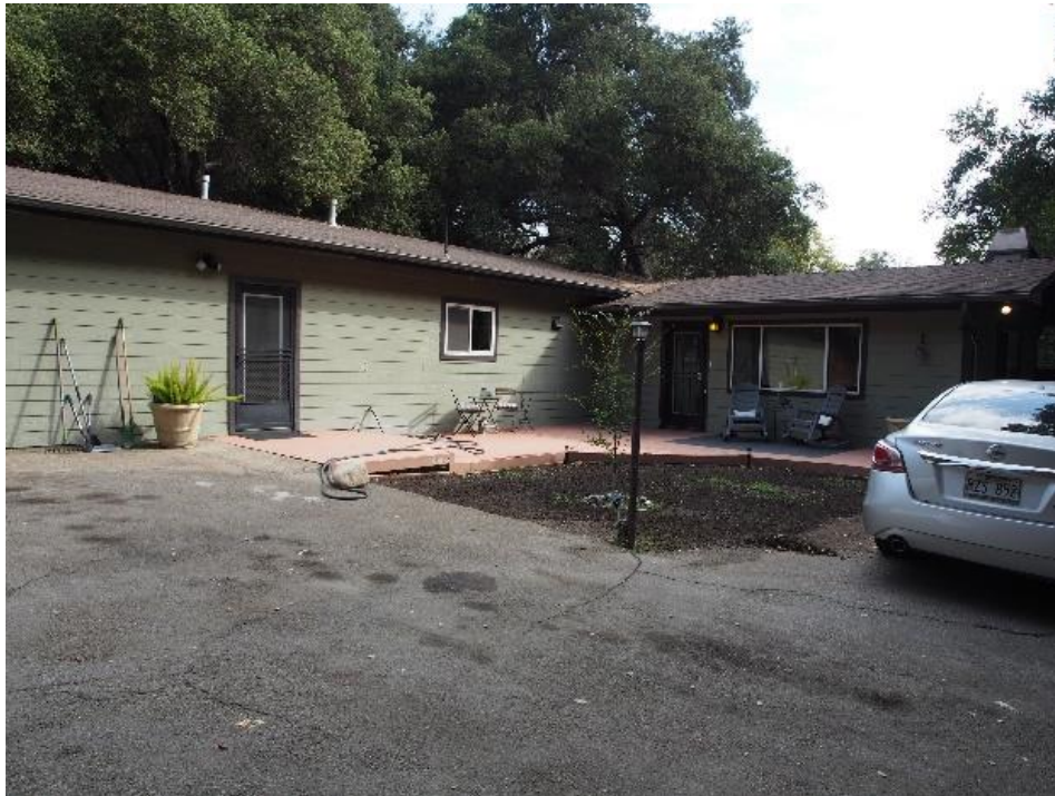
Photograph 36. Overview of main (southwest) elevation, view to northeast
