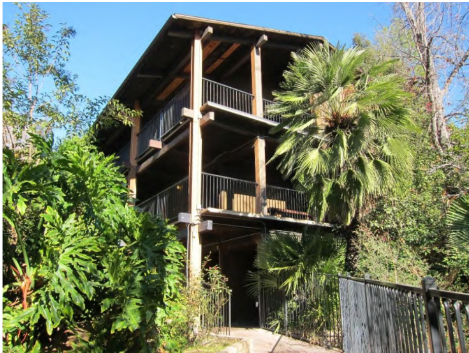
Photograph 18. Overview of south elevation, view to north
