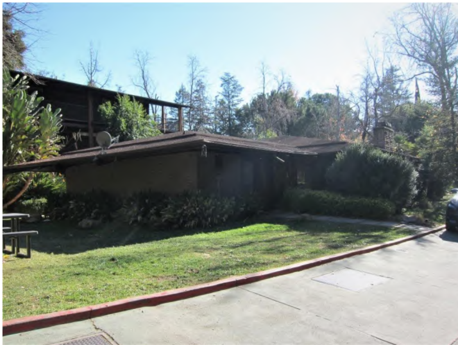
Photograph 22. Overview of north and west elevations, view to southeast
