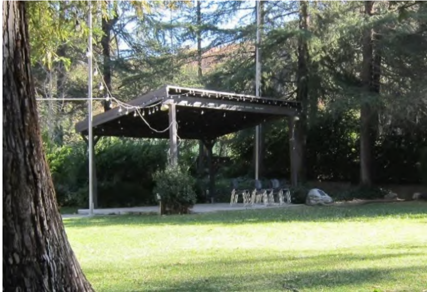
Photograph 9. Overview of gazebo, view to southeast
