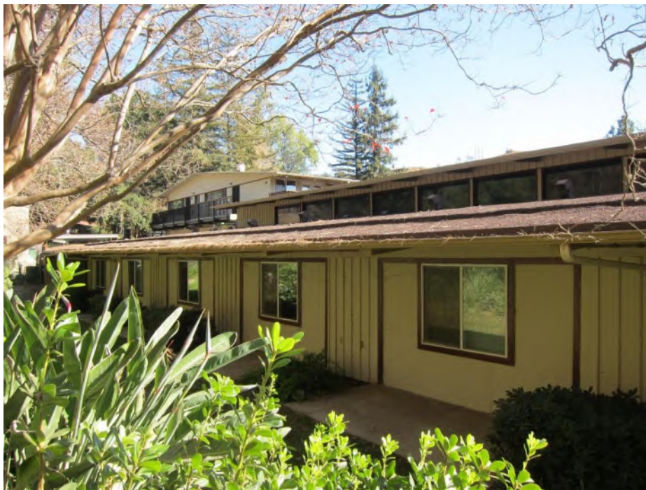
Photograph 31. Rear (west) elevation showing clerestory windows and replaced vinyl windows, view to northeast
