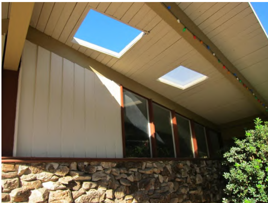
Photograph 30. Overview of roof openings and materials on front (east) elevation
