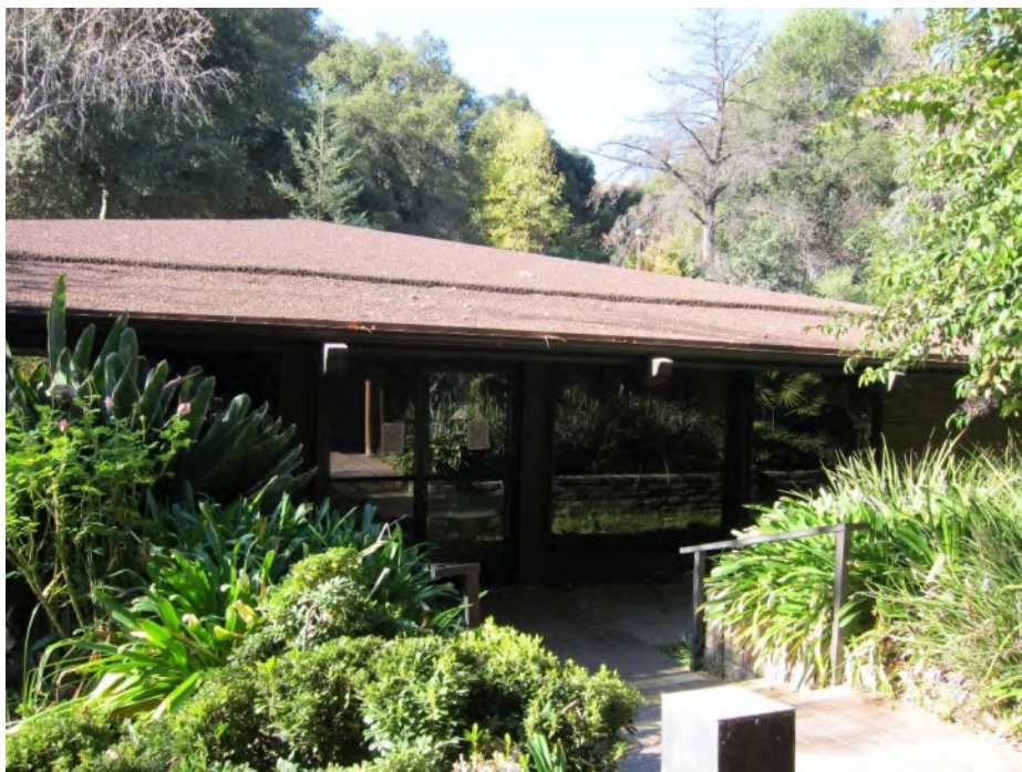
Photograph 20. Below grade entrance on the east elevation, view to west
