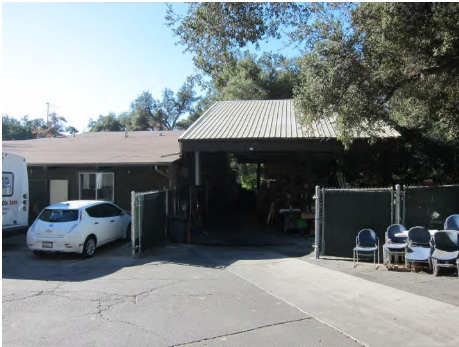
Photograph 7. Rear structure addition, view to southwest
