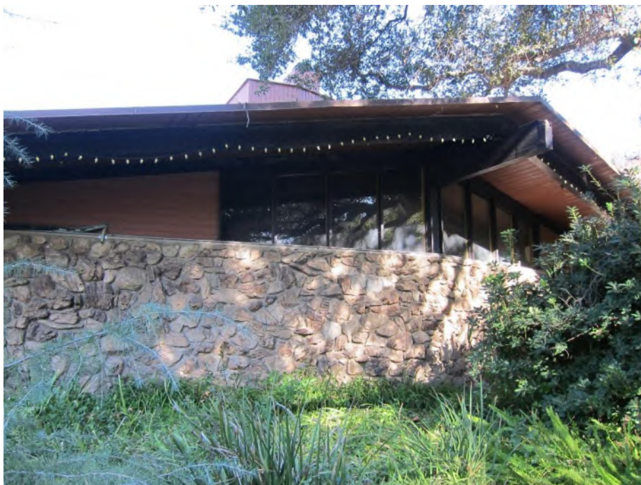
Photograph 13. Single-story portion of south elevation, view to northeast
