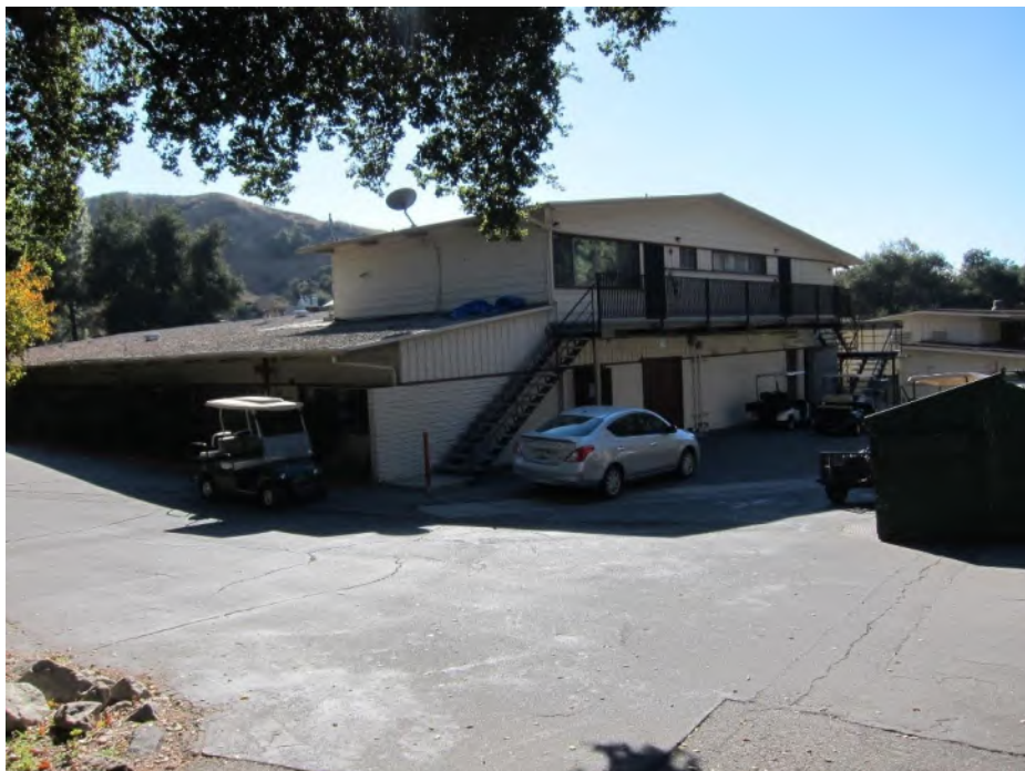
Photograph 27. Rear (west) elevation showing second story component, view to southeast
