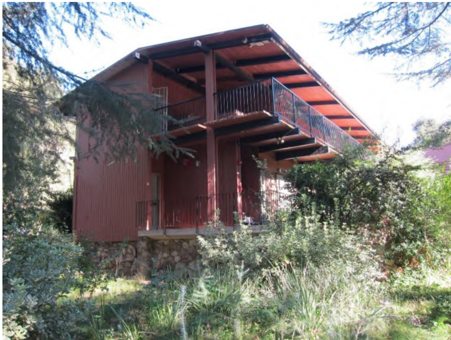
Photograph 11. Overview of south and west elevations showing side paneling, view to northeast
