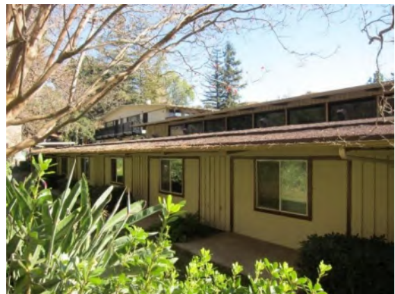
Photographs (from top): Main (east elevation), view to west; Overview of east and south elevations, view to northwest; Overview of roof openings and materials on front (east)
