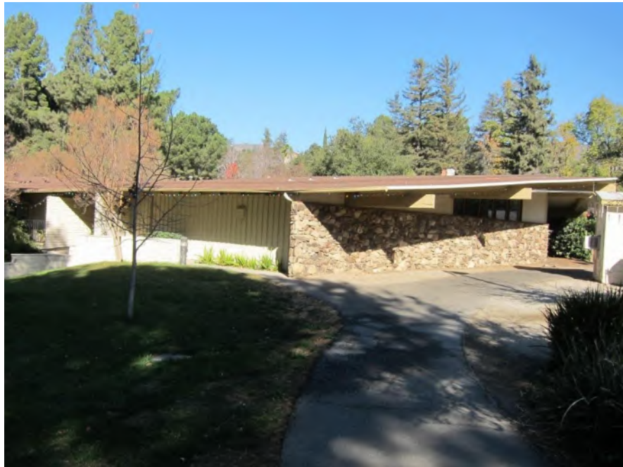
Photograph 29. Overview of east and south elevations, view to northwest
