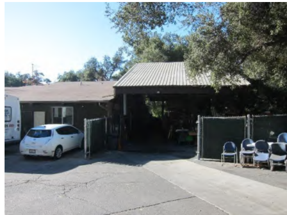
Photographs (from top): Overview of main (east) elevation, view to west; East elevation and partial view of slant roof south elevation; rear structure addition.
