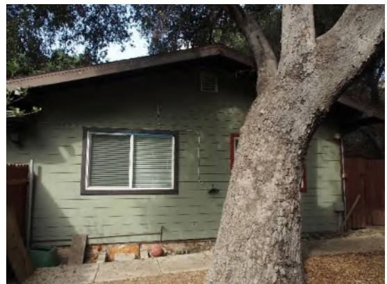
Photographs (from top): Overview of main (southwest) elevation, view to northeast; Rear (north) elevation showing French doors and shade structure, view to southwest; Overview of south elevation projection, view to north; and overview of east elevation, view to west.
