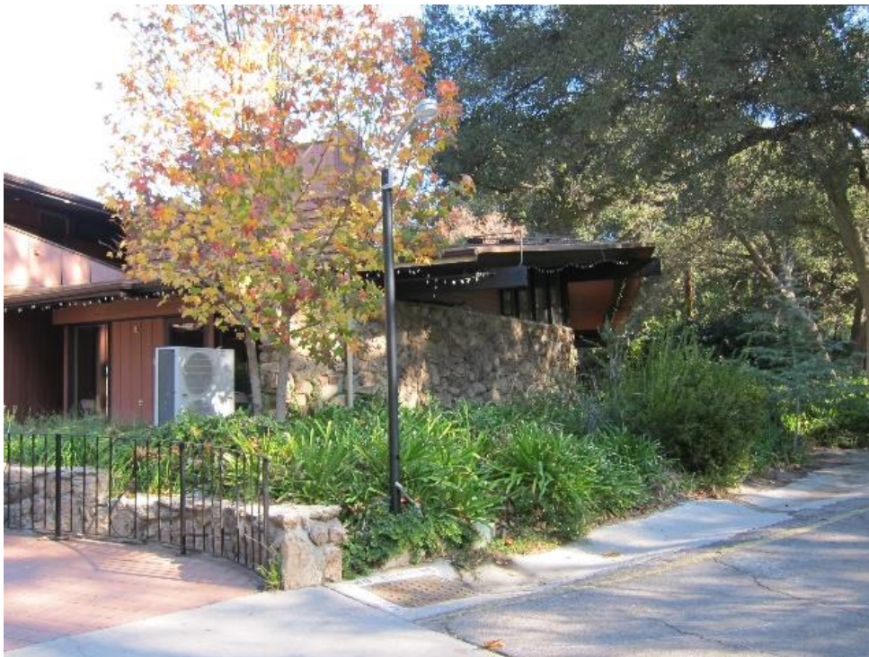
Photograph 15. West elevation, view to east
