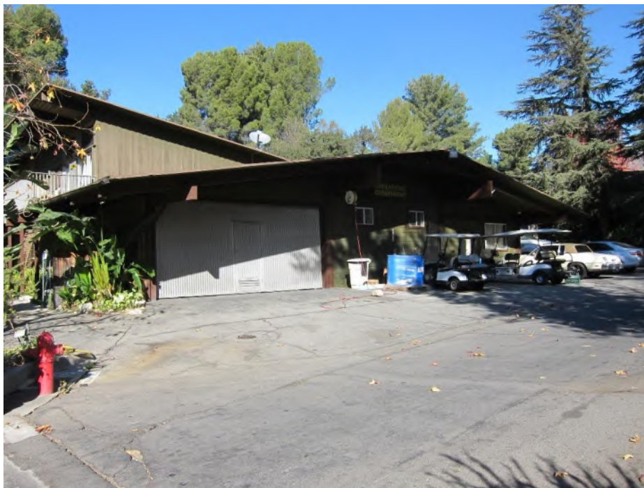
Photograph 6. East elevation and partial view of slant roof south elevation
