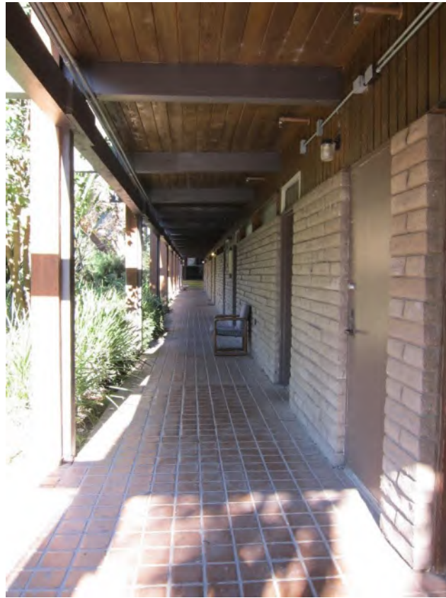
Photograph 17. Overview of ground-floor corridor, view to north
