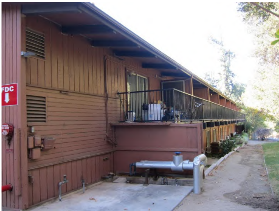
Photograph 12. Overview of rear (north) elevation, view to south
