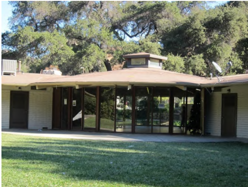
Photograph 32. Overview of rear (west) elevation showing circular lounge, view to east
