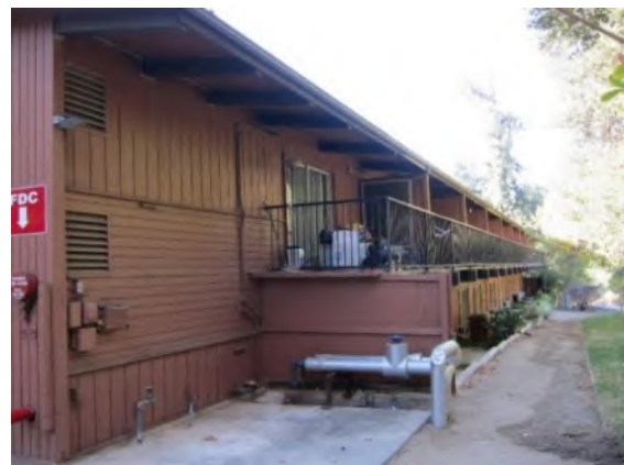
Photographs (from top): Overview of east elevation showing side paneling, view to west; Overview of south and west elevations showing side paneling, view to northeast; Overview of rear (north) elevation, view to south.
