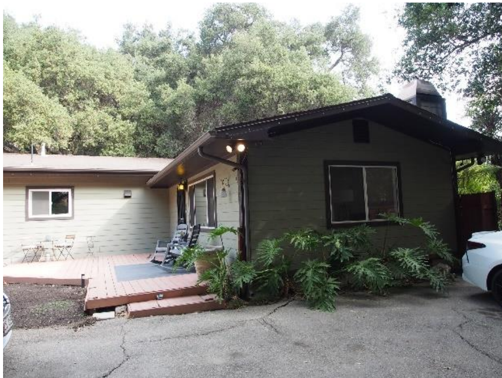
Photograph 38. Overview of south elevation projection, view to north
