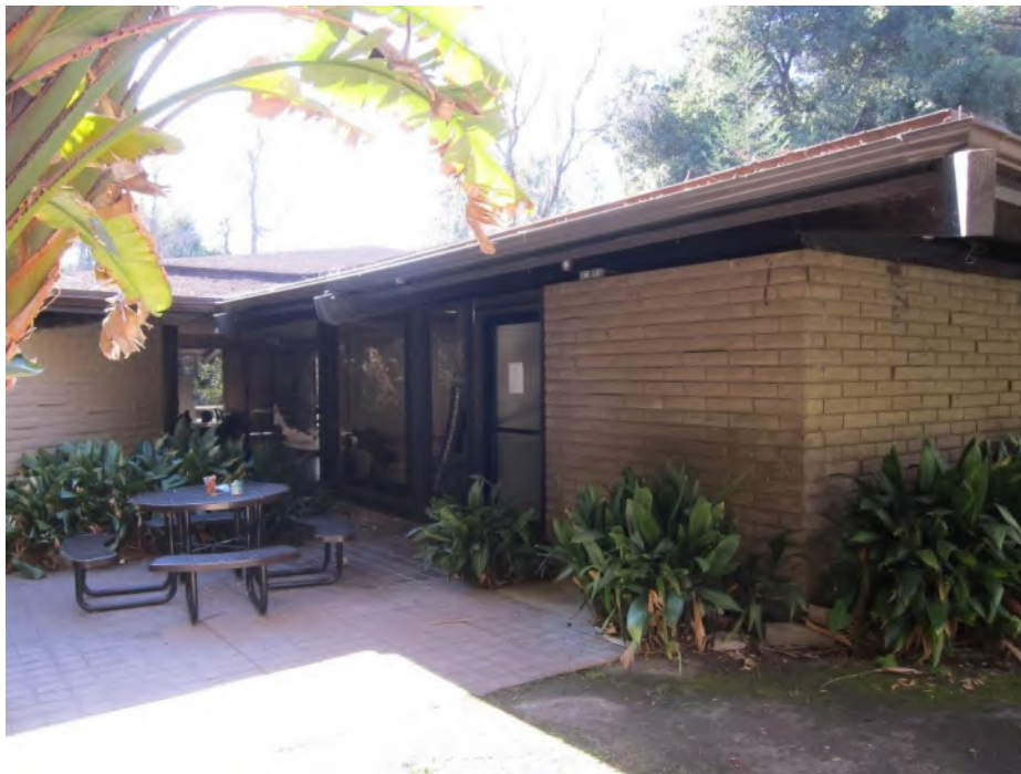
Photograph 19. Patio nook on the north and east elevations, view to southwest
