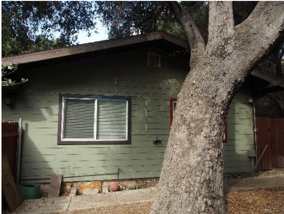
Photograph 39. Overview of east elevation, view to west
