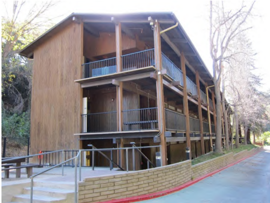
Photograph 16. Overview of north elevation paneling and patio area, view to south
