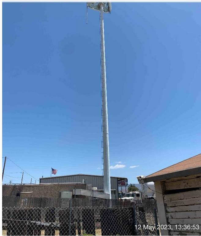
PHOTO 5- FROM WEST PROPERTY LINE
