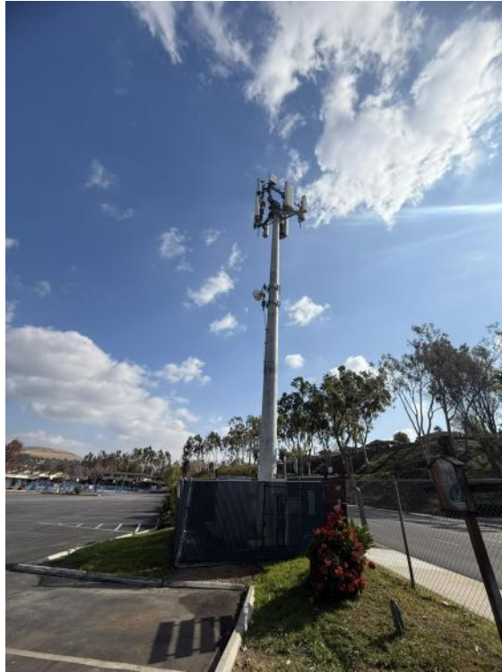
View from the West
