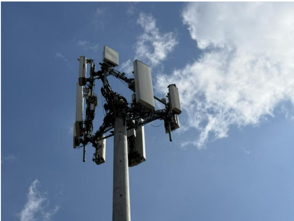
Antenna View from the West
