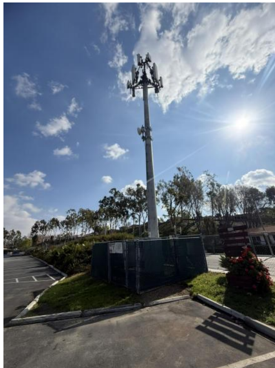
View from the West
