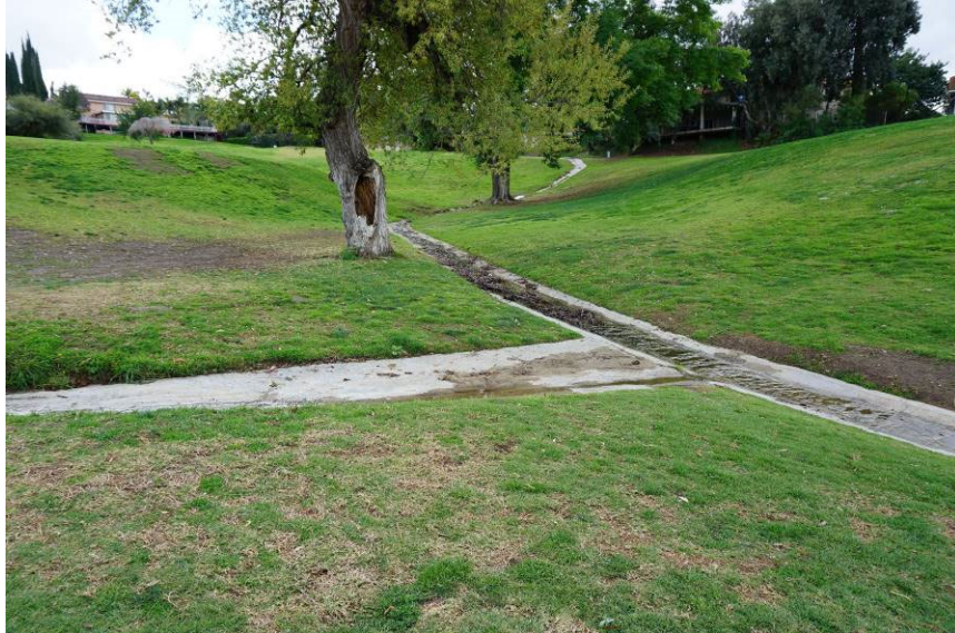
Figure 36 View of undulating concrete drainage ditches
