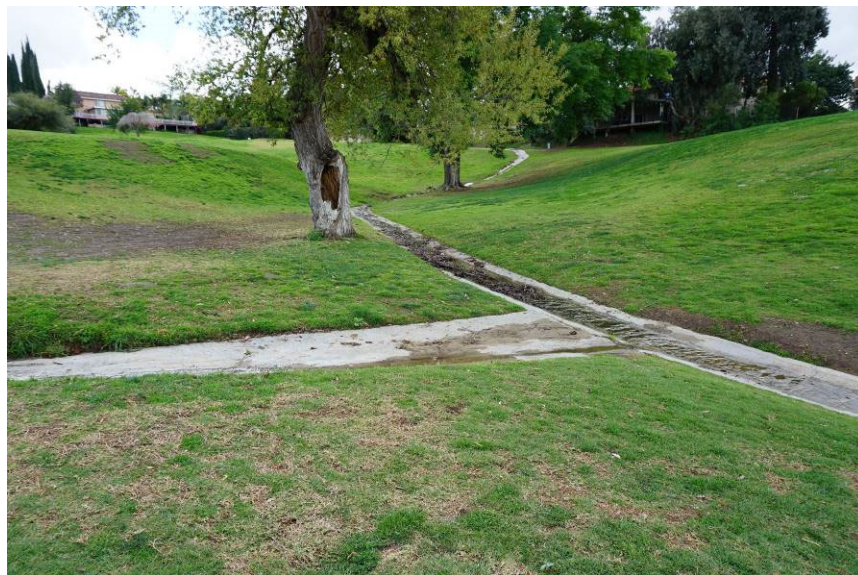
View of undulating concrete drainage ditches
