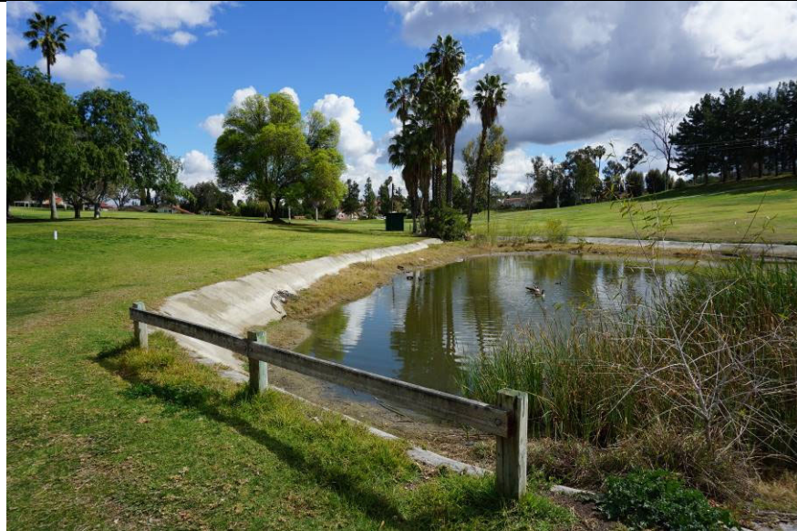
View of a concrete lined pond with simple wood barrier
