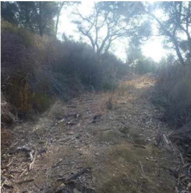
Figure 6. A 25.5 m-long by 2.5 m-wide area was graded and cut to provide access for heavy equipment. Photo taken 19 May 2021.
